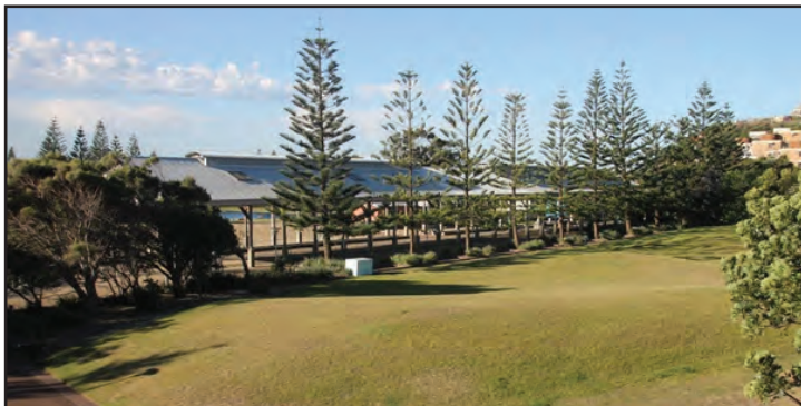
Part of the Newcastle Goods Yard and the carriage shed as they exist today. Image John Beckhaus
