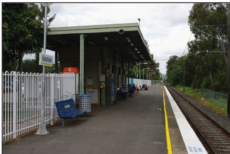
Schofields Station, looking towards Blacktown. The new, i.e. third, station will be about 800 metres distant. Image: Nev Pollard.
