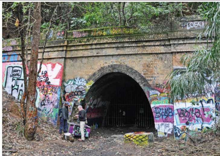
Above: The southern portal of Otford Tunnel as it appears today. The limited clearing out of the blockage done by the army in 1942, has resulted in the tunnel floor being partially filled. Image: David Taylor
