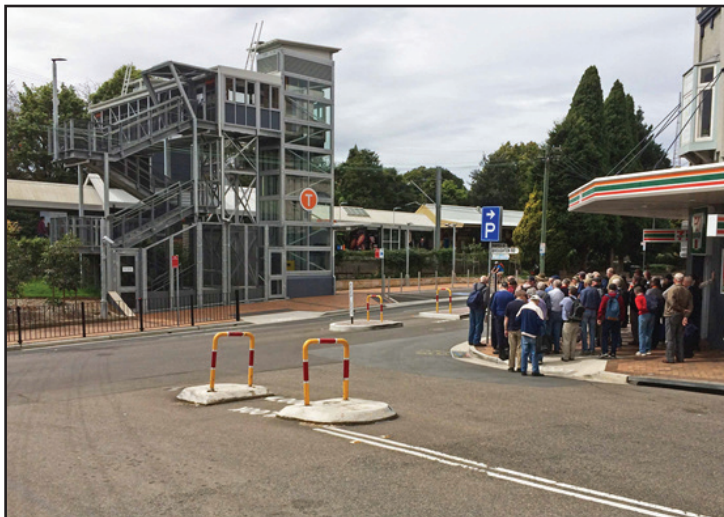
At the corner of Broughton Street and Hampden Road Artarmon, our group of about fifty gaze in wonder at the new lift facility with its overly large "T" sign. Image: David Taylor
