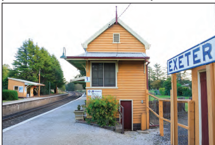
Exeter Signal Box on the northern end of the Up platform. The station building's awning can be seen behind. At the time of the crash, No.12 Fast Goods was reversing into the loop which became the Down Main with duplication.
