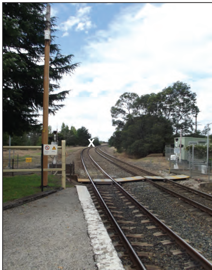
Looking north along the Up Platform. The white X marks the approximate crash location.
