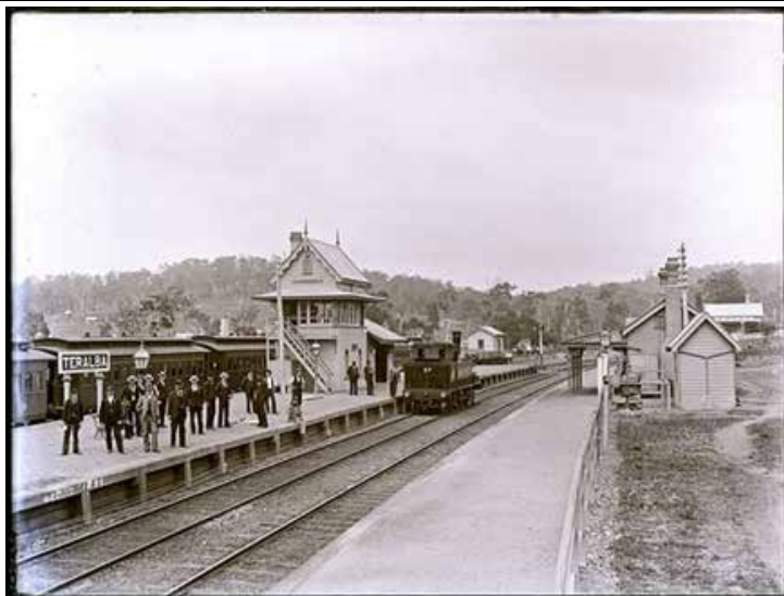
Teralba Station in 1899. The platforms and signal box on the left have now gone, and the Down platform on the right now forms part of an island platform with the 1982 Down main to its right. The Station Master's residence on the far right rear remains to this day.
