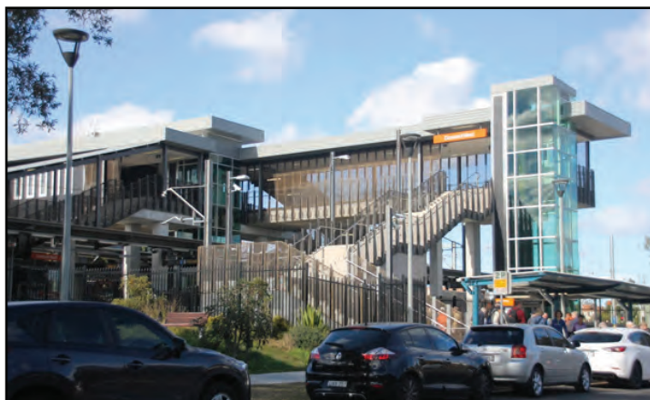
The large overhead station structure now at Concord West. Image: John Beckhaus.
