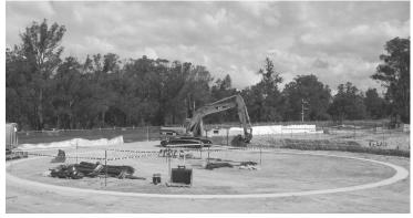
The circular concrete footing for the turntable's ring rail has been recently poured. The overhauled 105 foot turntable will be moved here and will present a raised 'stage' for displaying locomotives. The footings for the sector roundhouse are being formed-up on the right. The adjacent Loop Line has been slightly slewed to accommodate the width of the works. *Images by Ross Verdich*
