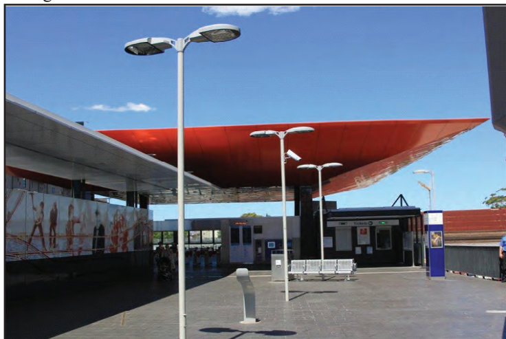
The new forecourt area and ticket barriers, under the cover of the large flat roof. Image: Peter Neve.
