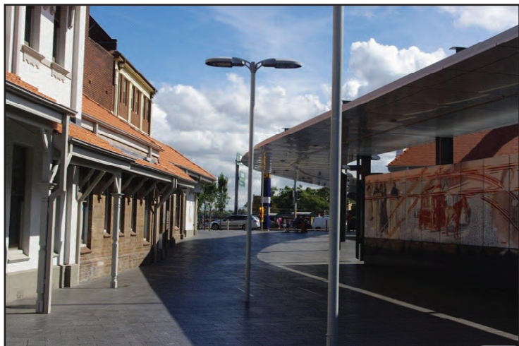
Newtown Station's forecourt, looking towards King Street. The restored former tram offices are on the left, and a large train and tram oriented mural is on the right. Image: Nev Pollard.
