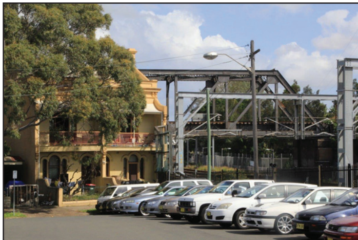
Above: A former railway residence at Sydenham which is now commercially leased. The recently demolished Station Master's residence was to the left, diagonally opposite this residence. Image: Peter Neve.
