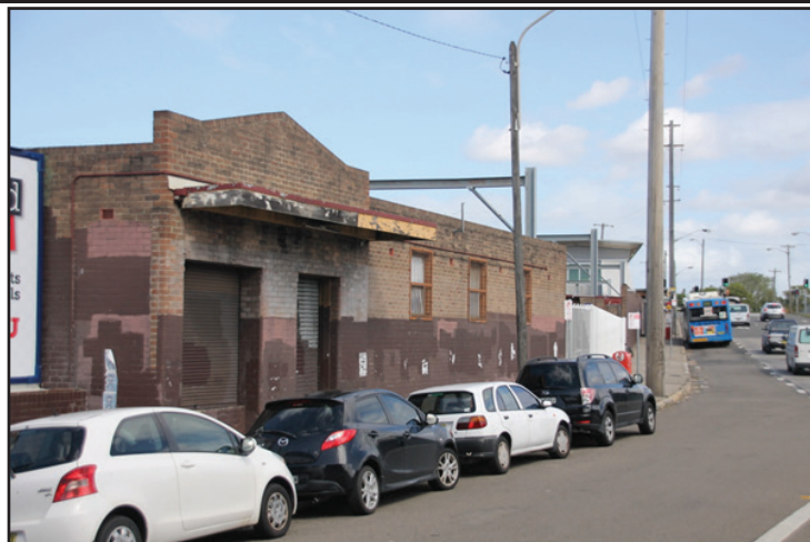
Above: The 1963 vintage former Parcels Office at Sydenham.
