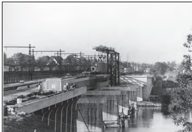
The second Meadowbank Bridge during construction in 1979. The floating crane is positioning one of the box girders onto the piers. The view is looking south towards Rhodes.
