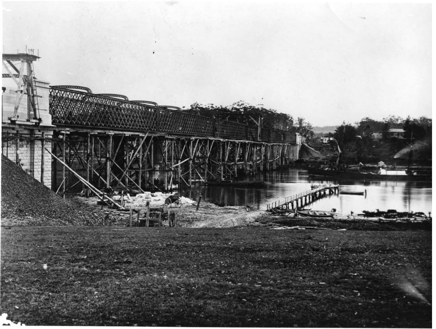
Image 8. Construction photos. The timber falsework used to support the ironwork until it was self supporting is well illustrated.
