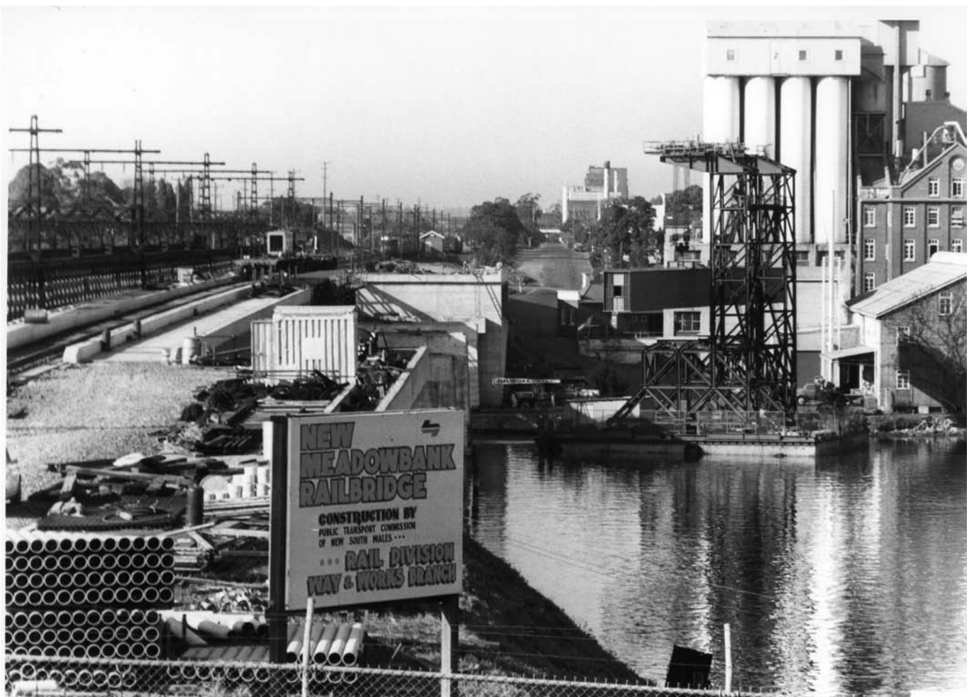
Image 12. The floating crane moves the girder to its final location.
