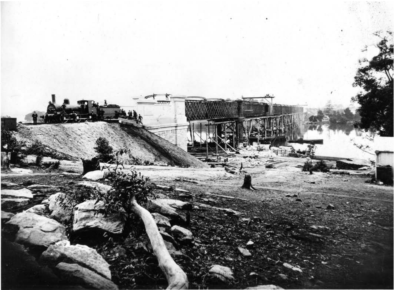
Image 6, 7. Construction photos. The timber falsework used to support the ironwork until it was self supporting is well illustrated.
