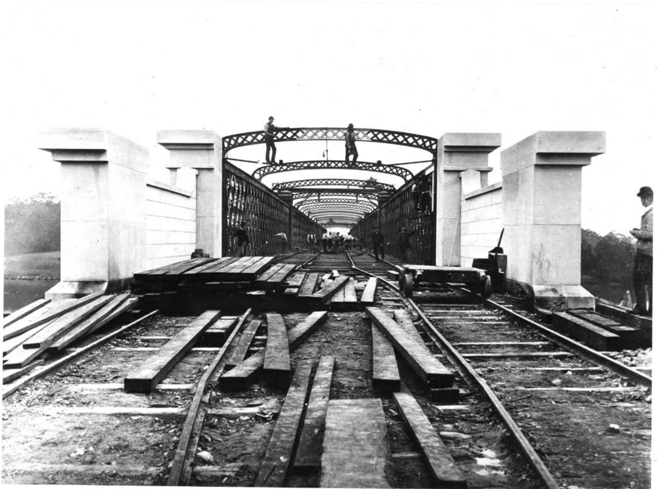
Image 6, 7. Construction photos. The timber falsework used to support the ironwork until it was self supporting is well illustrated.
