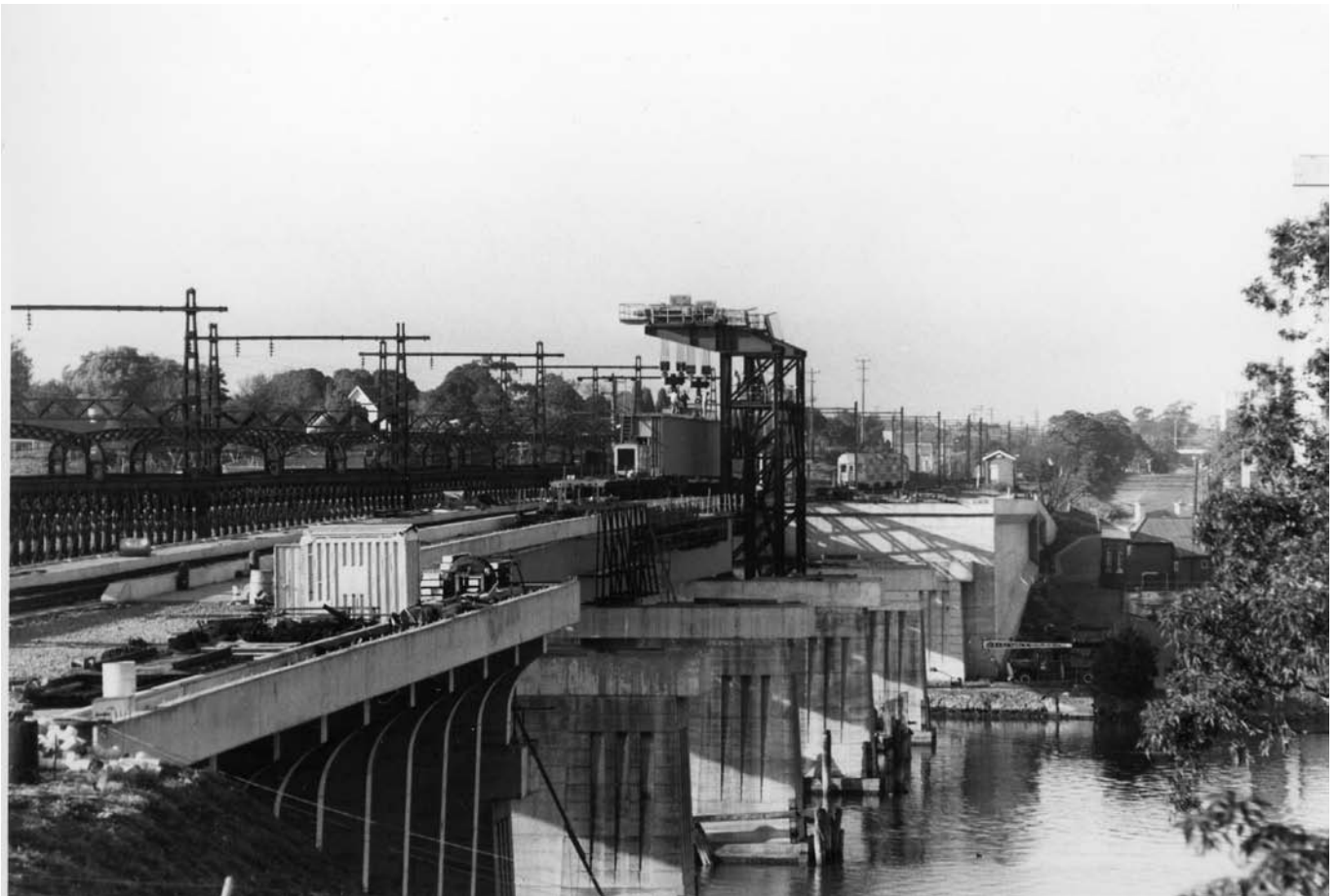
Image 11. Placing the box girders for the new bridge The floating crane has lifted the girder off rail wagons shunted onto already placed spans.
