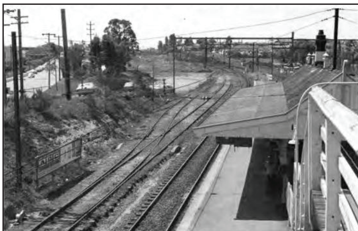
The Down loop and sidings servicing the industrial area of Regents Park c.1975, looking towards Lidcombe. This photo was taken by KT Groves and published in Bulletin No.520, February 1981.
