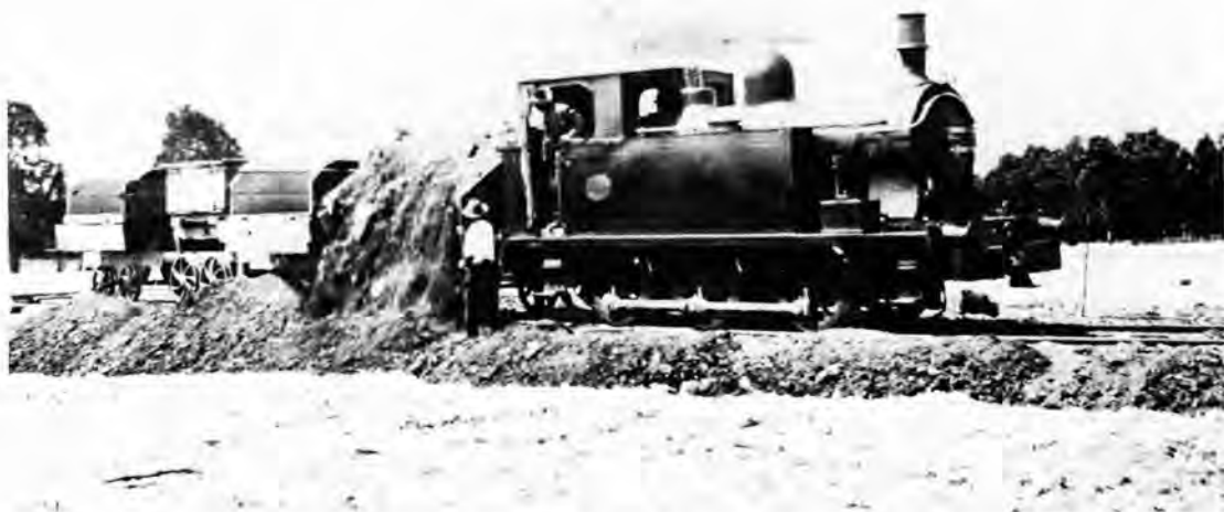
The Andrew Barclay locomotive shown at the head of a train of the early type of dump car was acquired by the Metropolitan Board of Water Supply and Sewerage in 1913. It was purchased from the Public Works Department, but ultimately one of six locomotives acquired for work at Potts Hill in the construction of the No. 2 Reservoir. These smaller dump cars proved too small for the work. (Photo: M.W.S. & D.B.)
