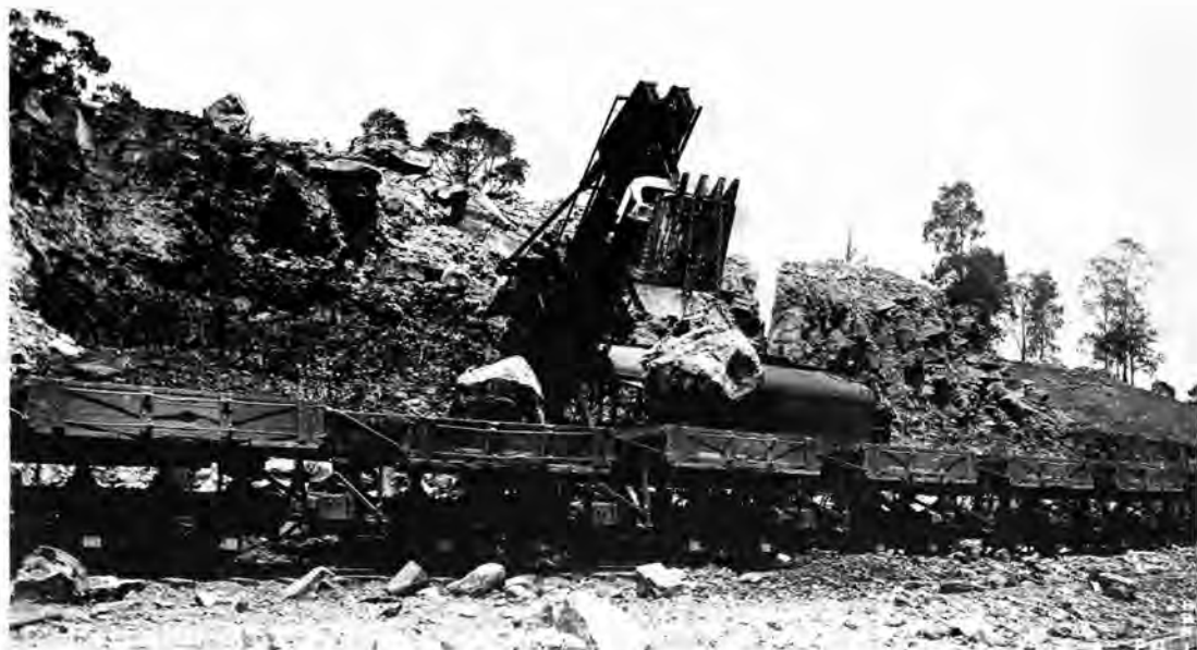
Bucyrus steam shovel loading rock by means of chain slings into a rake of dump cars on 24th January, 1914. (Photo: M.W.S. & D.B.)
