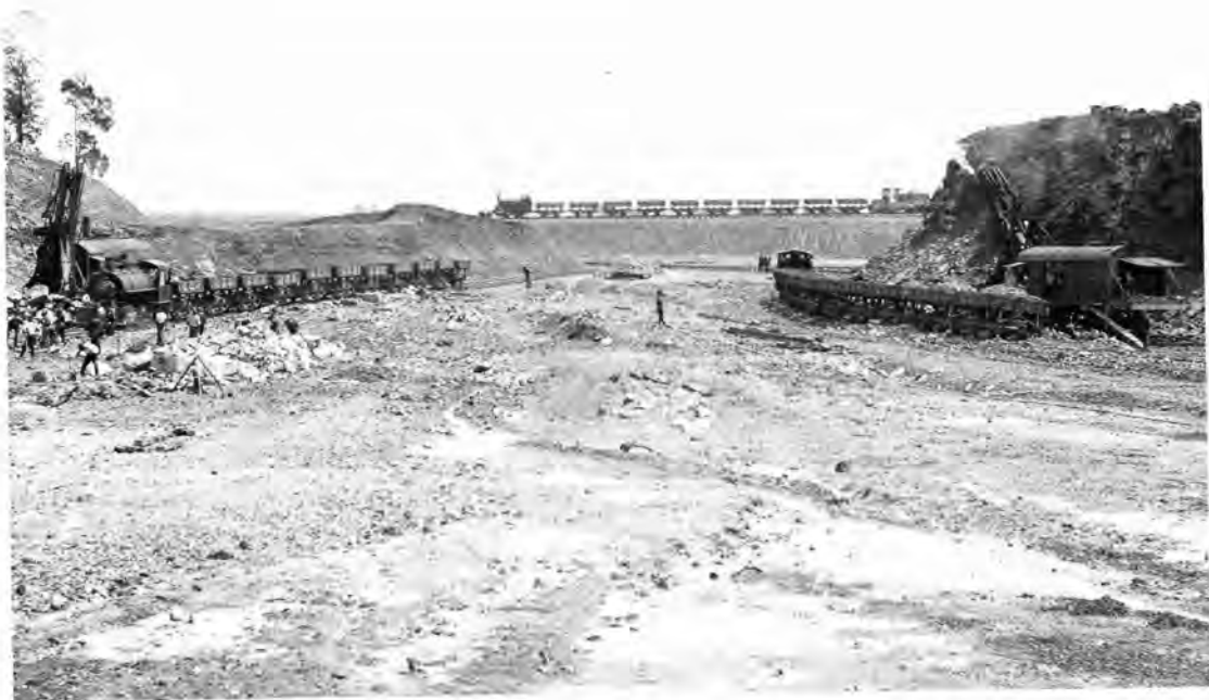
A busy scene with both the Bucyrus rail-mounted steam shovels at work during the construction of the second Potts Hill reservoir. In the background can be seen a Manning Wardle locomotive with Western dump cars and the spreader car operating. (Photo: M.W.S. & D.B.)
