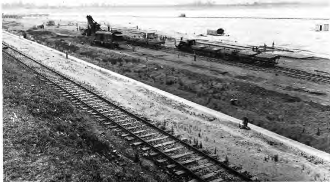
The reservoir had reached an advanced stage of construction when this photograph was taken, about 1922. One of the Manning Wardle locomotives is seen in the foreground with gravel for the concrete mixers. A Bucyrus steam shovel is still at work removing spoil from the reservoir floor. One of the Vulcan locomotives is seen in the right background with its rake of cars. (Photo: M.W.S. & DB.)
