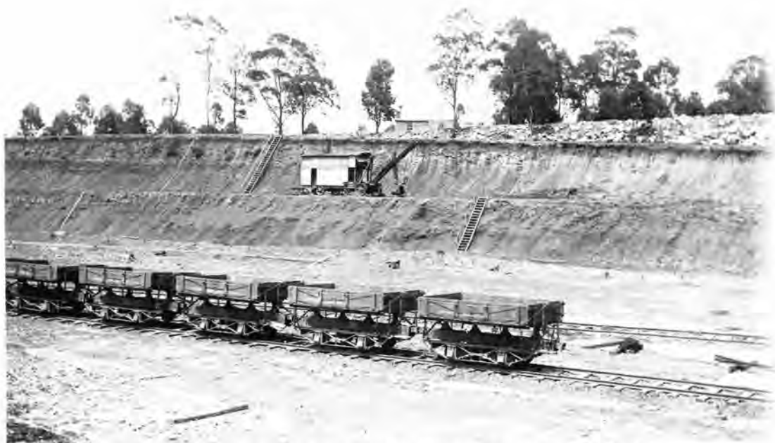
The Ruston Proctor steam shovel is seen on an intermediate level, with a rake of Western dump cars on the floor of the reservoir. At this stage a good idea of the amount of excavation necessary in a large civil engineering project can be obtained, the date would be about 1917-18.
