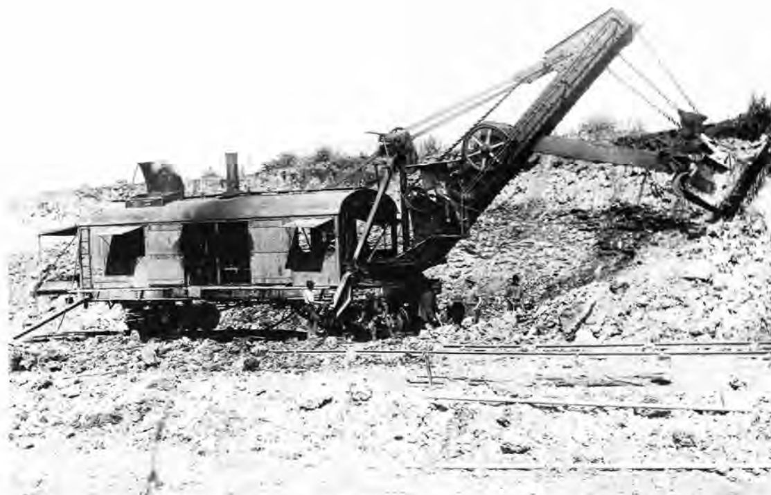
A Bucyrus Steam Shovel at work in 1915. Three men were necessary to work the shovel. A Fireman tended to the needs of a locomotive type boiler at the rear of the machine, the cylinders of the engine can be seen in the centre opening of the body. A Driver in the front of the shovel controlled the luffing (or side to side movement) of the boom, and also controlled the forward and backward movement of the shovel up to the working face. On the boom can be seen a further small cabin, in which was situated the Boom Operator. His functions were to control the run in and run out of the shovel arm, and also to release the bucket latch as required. Only the forward bogie of the shovel was powered.
