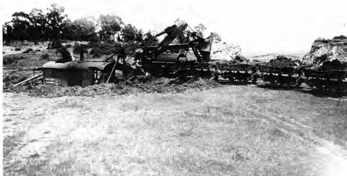
A Bucyrus steam shovel is shown working in a cutting, while loading a train of the later Western dump cars in 1914. The train is hauled by one of the Vulcan locomotives. (Photo: M.W.S. & D.B.)
