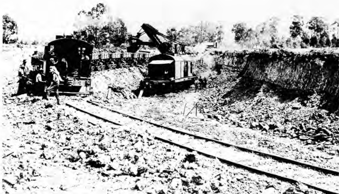
Men at work in rather heavy going following wet weather. In the foreground is a Vulcan locomotive with its loaded cars of spoil. The steam shovel is a Bucyrus which is rail-mounted. In the background at a higher level is seen the narrow-gauge Fowler locomotive.
