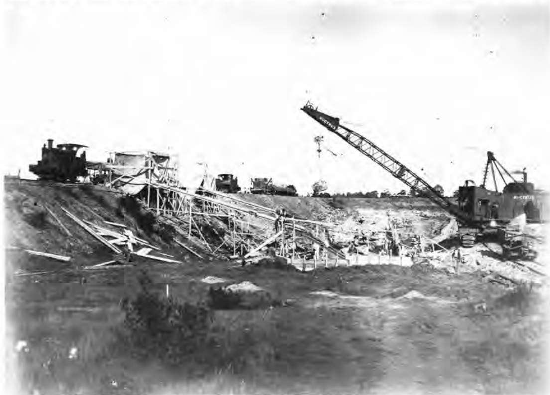
This view shows the fourth steam shovel which was acquired in 1915. It was a Bucyrus drag line bucket engine and ran on tracks, rather than rail-mounted, and is seen helping with the concrete work in 1921. On the wall of the reservoir can be seen two Manning Wardle locomotives, and the Vulcan on a train of dump cars and the spreader car.
