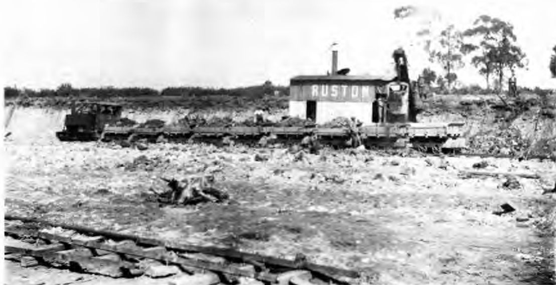
This photograph shows a train of the smaller (earlier) dump cars. The cars are part of the 2'6" narrow-gauge system used by the Board. The locomotive is a Fowler 0-4-0T type of uncertain origin. The presence of the Ruston Proctor steam shovel dates the photograph to 1914. (Photo: M.W.S. & D.B.)
