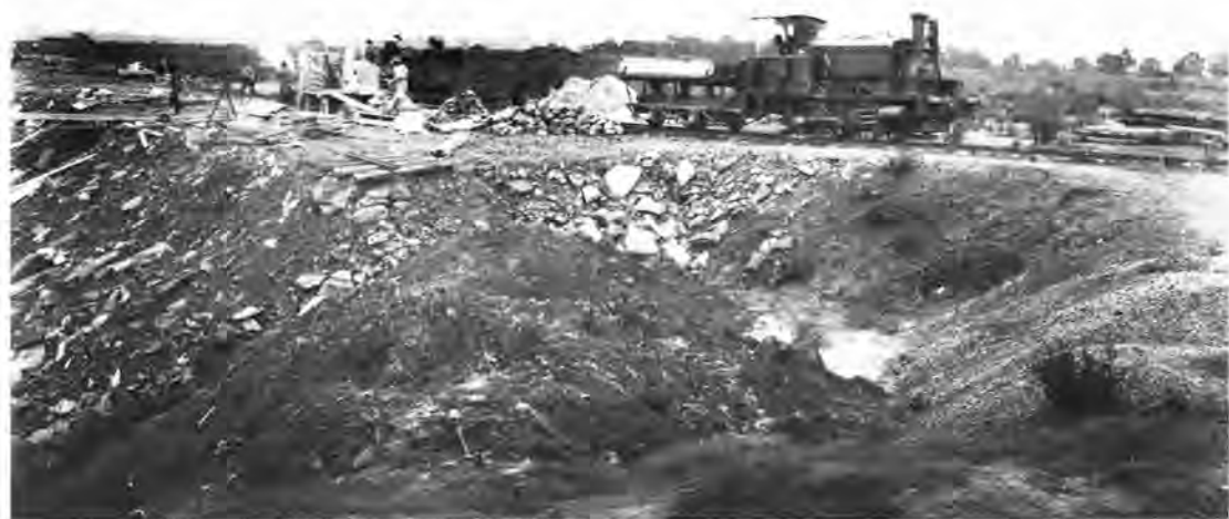
A Manning Wardle with its train of Western dump cars, bringing sand to the concrete mixers, about 1921. (Photo: M.W.S. & D.B.)
