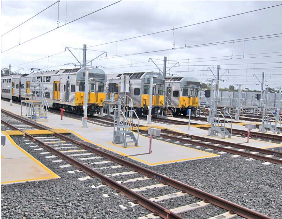
Part of Leppington Yard on 21 March 2015. The trains are on sidings 8, 7 and 6. Note the short platforms that allow easy access to the trains by the crews. John Oakes IMG_1364.
