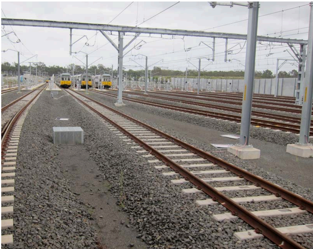
Part of Leppington Yard on 21 March 2015. The trains are on sidings 8, 7 and 6. Note the short platforms that allow easy access to the trains by the crews. John Oakes IMG_1364.
