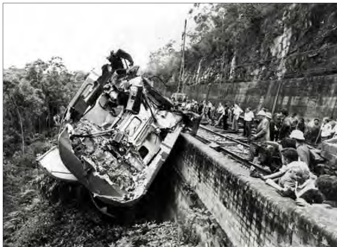
On 16 January 1976, 21.30 Sydney–Mount Victoria Interurban train stalled outside Glenbrook tunnel and was hit in the rear by 4622 hauling 20.20 goods, Darling Harbour–Orange at 22.45. Double-deck car DCF8004 is seen here being rolled over the embankment in an effort to clear the Main Western Line.
