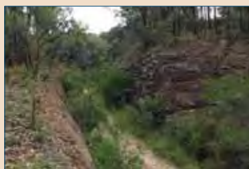
The scene along the single track 1892 deviation. Lapstone Safety Siding was a short distance further on.
