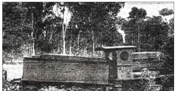
In January 1926, 5365 and a wagon ran away from Falconbridge as a result of a broken coupling and the driver falling out of the cab. The train reached an estimated speed of fifty miles per hour through Springwood. It was stopped by being routed into the 'head-in' refuge siding at Blaxland Junction. This Siding Formed Part Of The Original Main Line.
