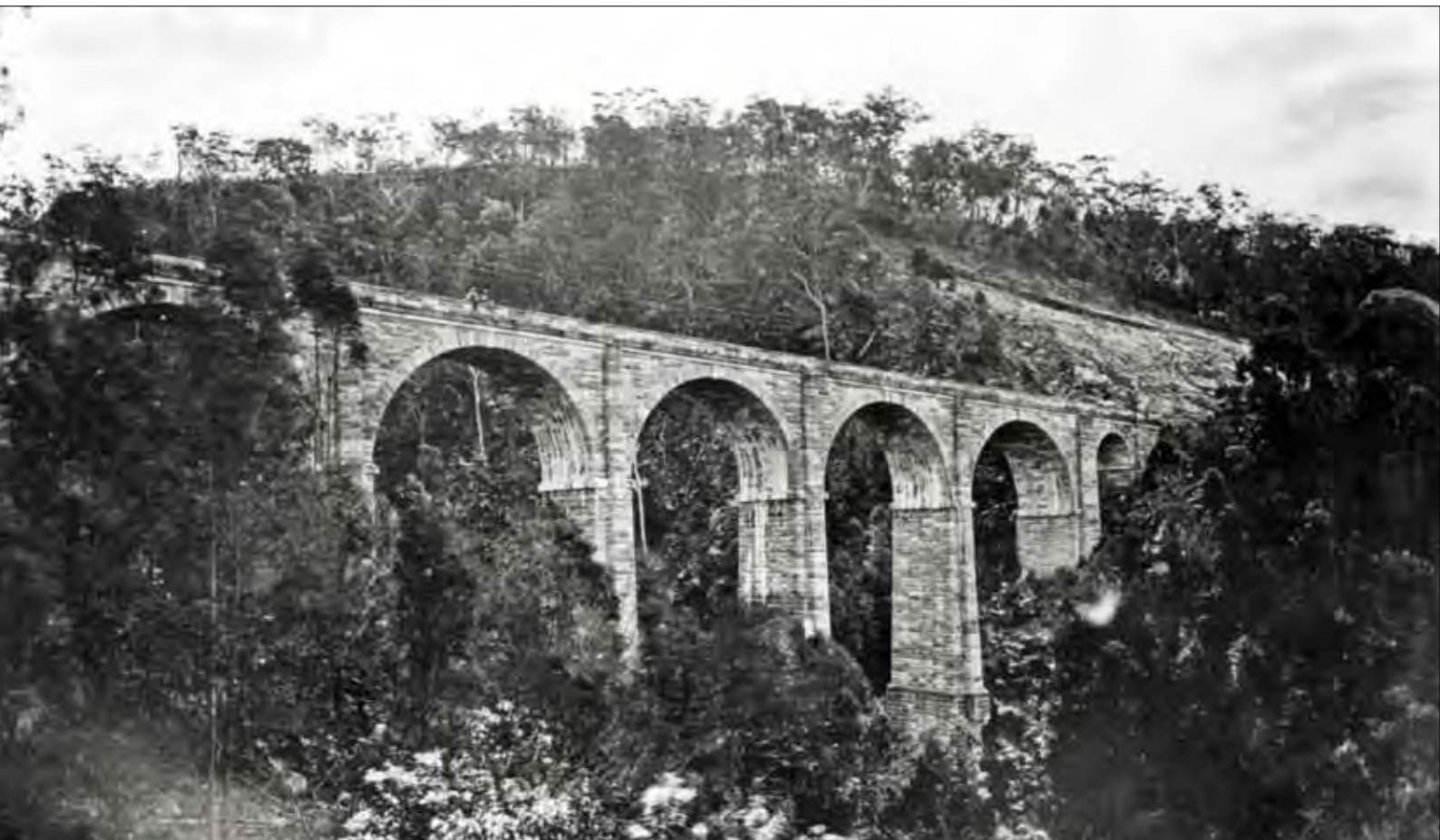
Knapsack viaduct . The first Knapsack Block Post was located south (left hand end of the photo). The second site of Knapsack was located about four hundred yards to the right of the bridge. The Down Refuge Siding ended at the top of the gully on the extreme right of the photo. The bridge was widened when taken over as part of the Great Western Highway. N Thorpe collection ARHSnsw Railway Resource Centre 23764a
