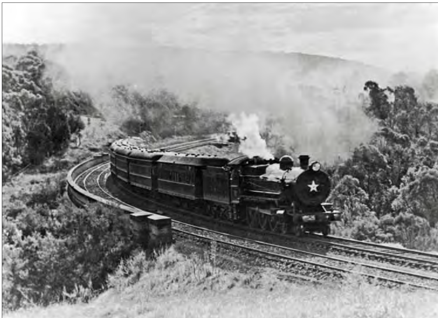
3526 hauling the Caves Express over the new Knapsack Viaduct on Lapstone Hill.
