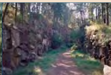
The cutting along Top Road between the junction with Middle Road and Knapsack St Glenbrook. Note the vertical bore holes where explosives were added.
