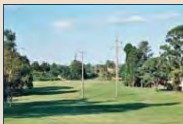
The double track deviation left the original single line just east of Russell St Emu Plains. This was the location of Nepean Jn. The image is taken on the site of the original track. RailCorp's feeder line follows the location of the old track at this point.
