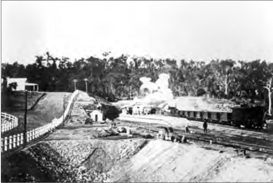
The new Glenbrook Station on the second deviation. This view was taken from the west, and the short goods siding is in the foreground, while the recent earthworks and the positioning of the ballast train in the wrong direction suggest that work may have still been in progress.
