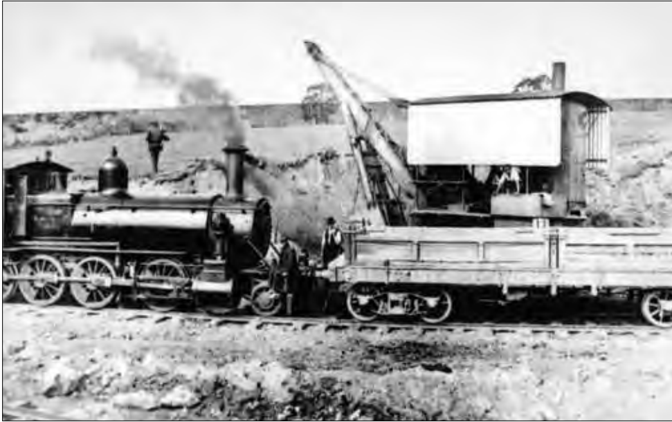
A Ruston steam navy appears to have been used here for the first time in NSW. This is a 2-8-0 tender type locomotive, one of the Baldwin-built 131/J131/X10/Z28 Class locomotives. It would have been on the Glenbrook Gorge deviation construction branch.
