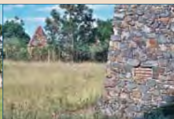
The old gatekeeper's cottage marks the location where Bathurst Road (now Mitchell's Pass) crossed the original single line. The present line is located behind the cottage with the bridge over the former highway to the left. On the right is the John Whitton memorial.
