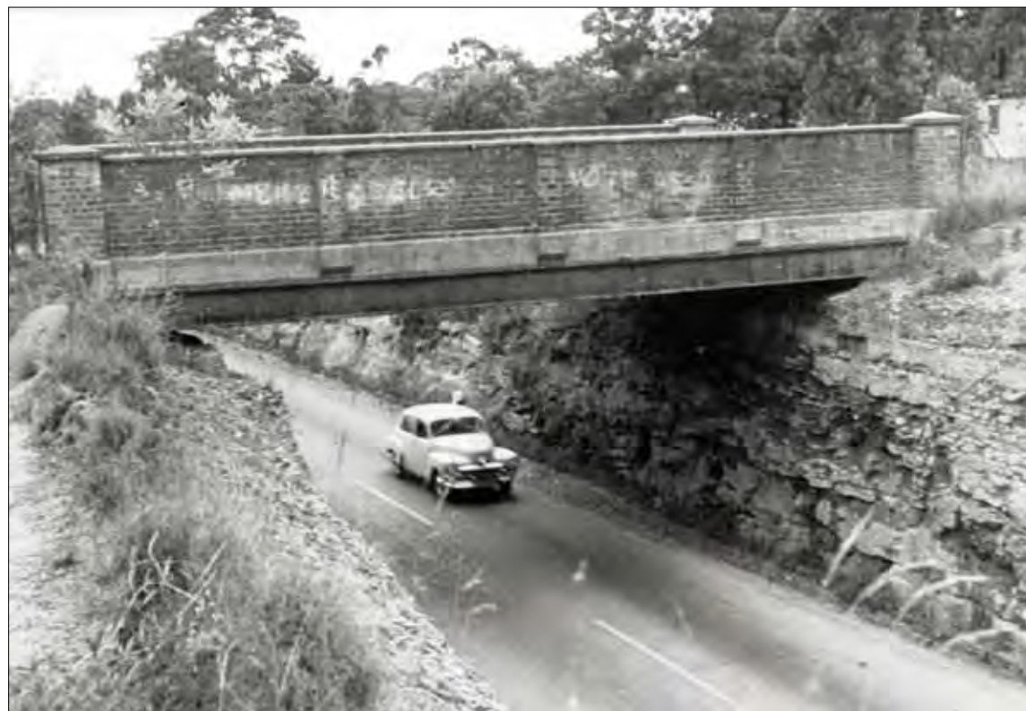
The Great Western Highway took over the old rail formation from about the present RAAF base to Blaxland. This photo is taken just west of the site of the first Glenbrook. The bridge and cutting lasted until the early 1980s when the highway was widened to four lanes and a new roadbridge was constructed.
