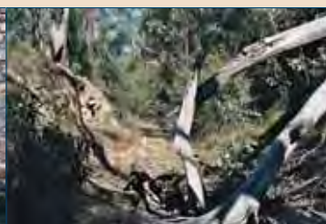
A scramble through the bush at the northern end of Knapsack bridge will reveal the end of Knapsack Down Refuge Siding. The buffer stops were located a few metres further on at the top of Knapsack Gully.
