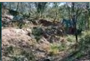
The scene at the end of Top Wing. The reader will note two formations. The lower was abandoned after the runaway of 22 March 1886 in favour of the top formation that was regraded to 1 in 33 against arriving trains.
