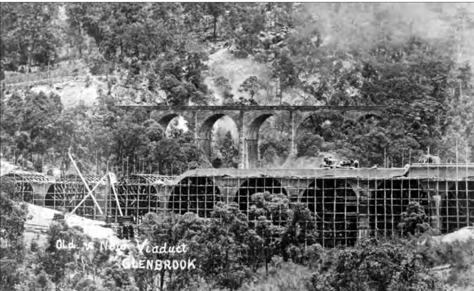
Old Knapsack Viaduct with new viaduct under construction circa 1911. N Thorpe collection, ARHSnsw Railway Resource Centre 23764b
