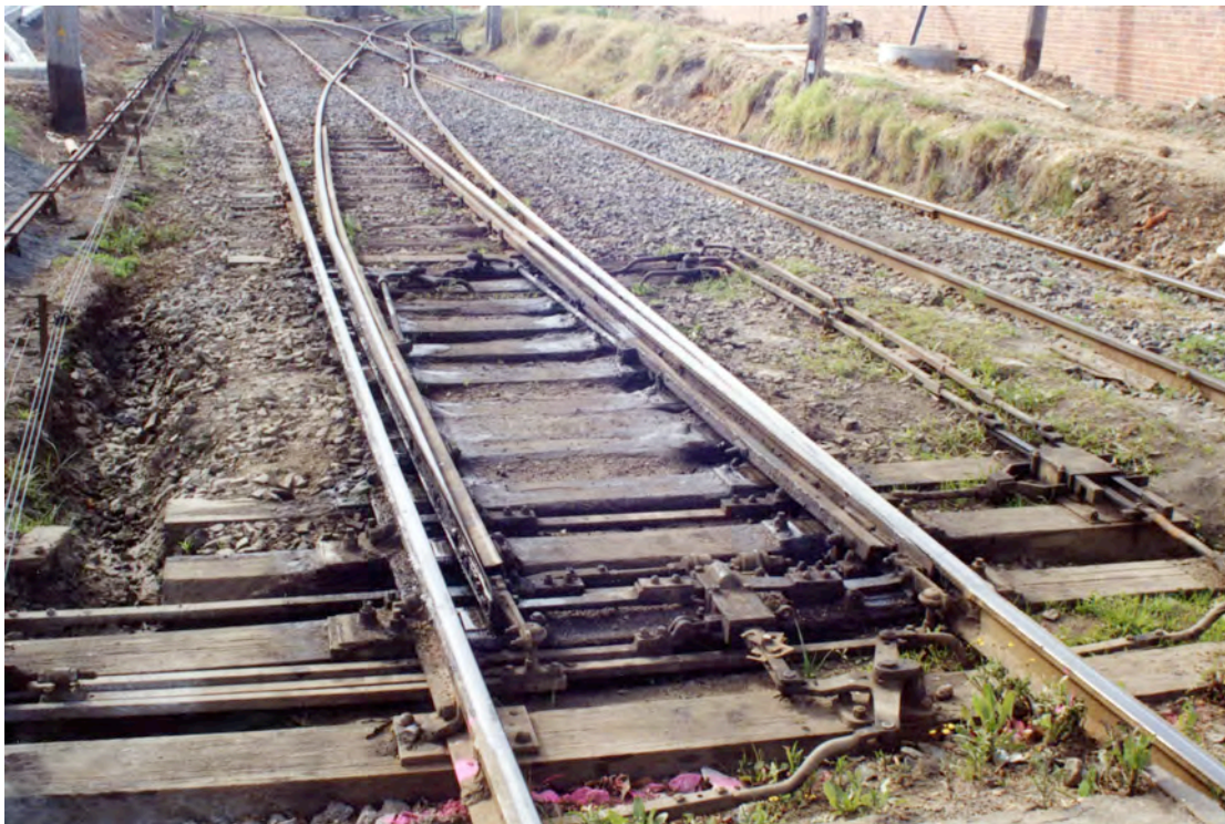
The junction for the Sandown Line. Note the single slip in the Up Carlingford line. ARHSRRC 106795
