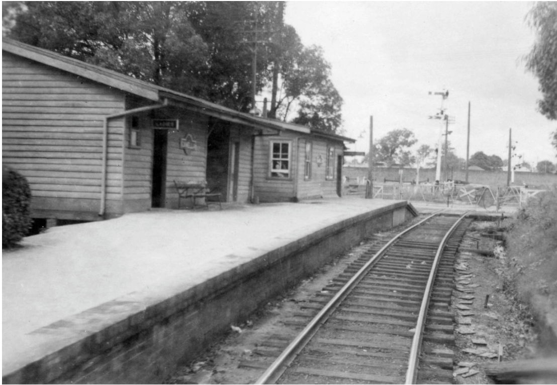
The buildings on the Camellia Station platform and the Grand Avenue level crossing with the hand operated gates. The signal on the Sandown Line that protects the junction is behind the pole in the right background. ARHSRRC 100681.
