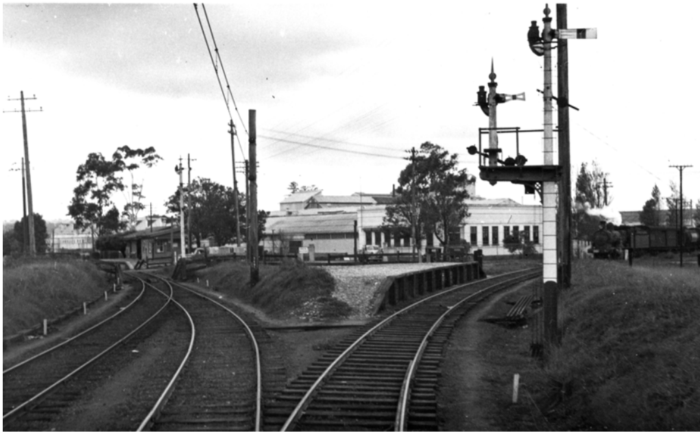
The first Hardies Platform was close to the junction. Camellia Station is in the left background. Note the wrong road signal that allowed trains from the Sandown Line to use the Down Carlingford line if the Up line was occupied by race trains (or the ambulance train during World War II. ARHSRRC 010028
