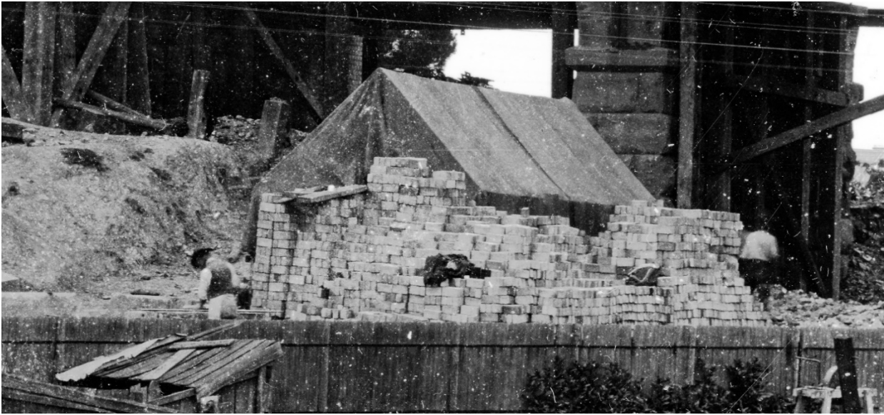
Figure 6 The bricks from the old bridge were evidently salvaged and cleaned for re-use. RRC 432464B
