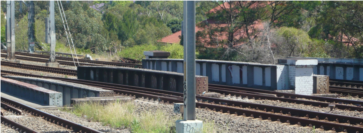
Figure 19 Viewed from Lewisham platform the markedly different sizes of the girders of the Suburban bridge is obvious. The left most girder of the 1886 bridge, then the three of the modified 1892 bridge and then the girders of the 1927 bridge. The three girders seem to be heavily cambered, but this may be partly an illusion created by the extra plates in the flange at the middle of the span. Bill Phippen photo.
