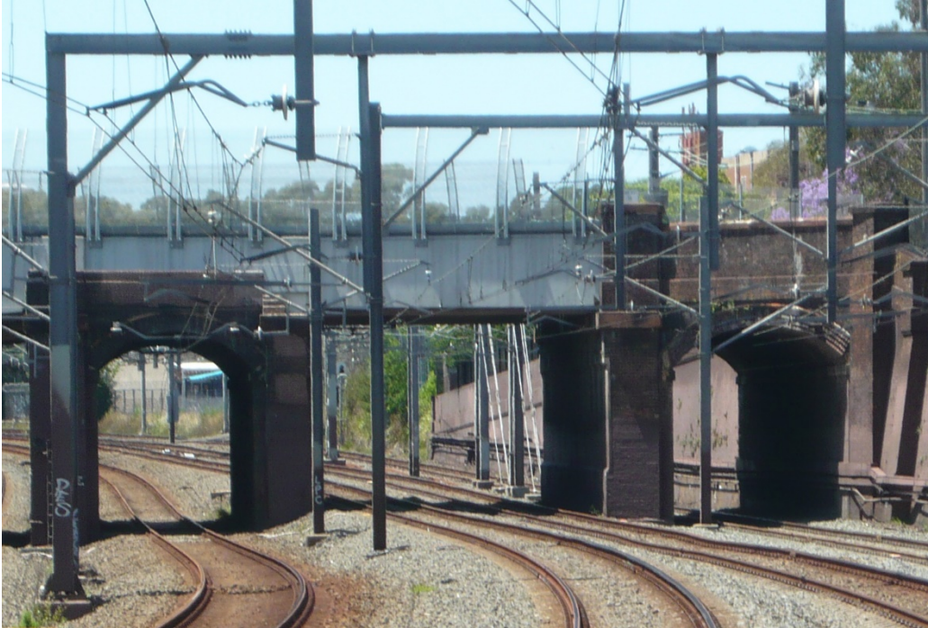
Figure 24 A distant view of the skew brick arch under West Street Lewisham, Bill Phippen Photo
