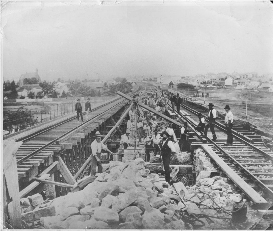
Figure 4 One track has been slewed into its final location, while trains run on the new bridge temporarily supported away from its final alignment. Once the masons have removed the old bridge, the trusses will be slid into their final location. RRC 34497
