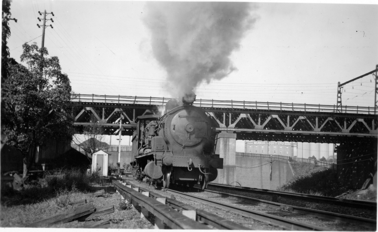
Figure 15 The Mainline Warren Truss bridge. In 2018 this 1927 span is the oldest superstructure component remaining over Long Cove Creek. RRC19269
