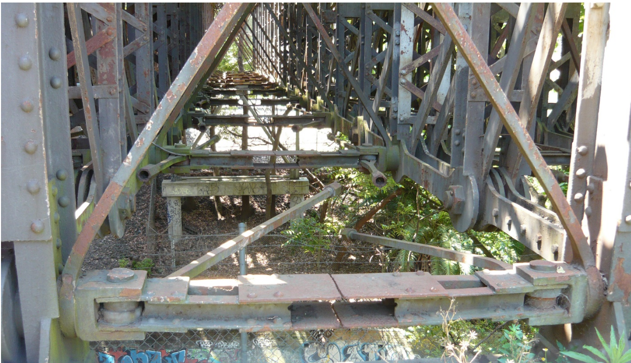
Figure 12 When track centres were widened the straight across members of the bracing between the two tracks were clearly cut and lengthened. The diagonals do seem a little more bent than the corresponding members between the trusses directly under the tracks. The large "C" shaped bracket to which the strut is pinned may be a nut on the end of the pin of the joint. Bill Phippen photo
