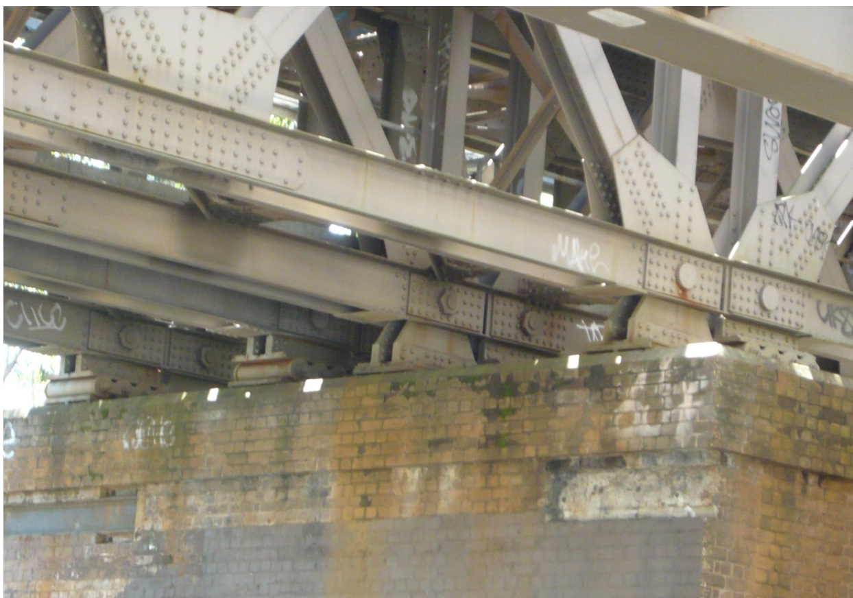
Figure 13 The bearings under the Warren trusses. The nearer pair are fixed and at the Sydney end of a Down truss and the moving bearing is at the Parramatta end. The farther two are rolling bearings and are at the Sydney end of the Up track. Bill Phippen photo
