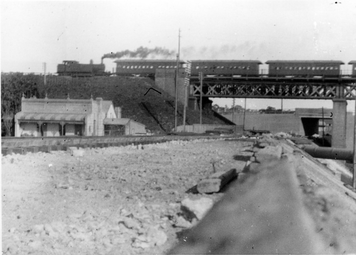
Figure 14 The lattice girders, before they were obscured by the later mainline bridge. RRC18356
