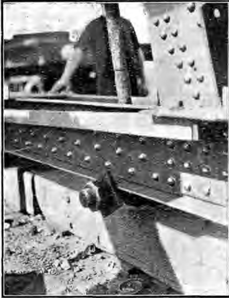
A "Close-up" of a lift into position.
