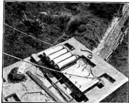
Rollers and Bed-plates which carry the ends of the spans, the former allowing for expansion and contraction of the steel through temperature variations.
