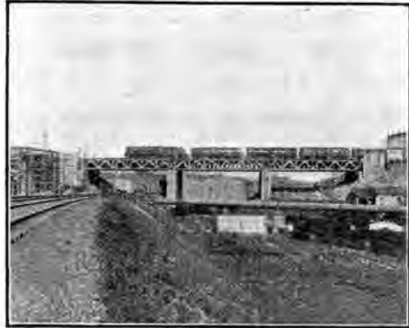
Lewisham Viaduct from Parramatta-road.
