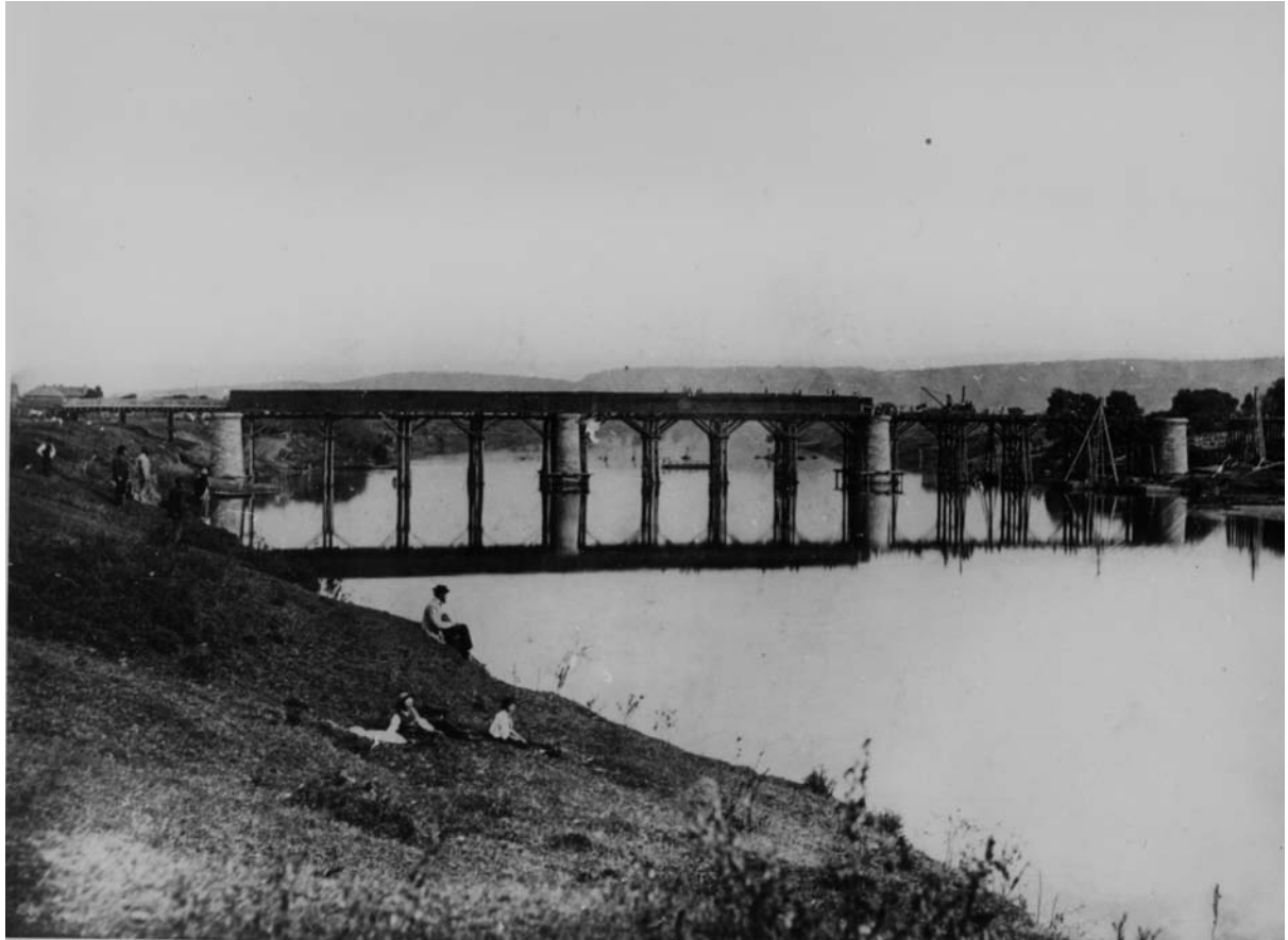
Photo 34277. The method of assembling the ironwork on timber staging is evident in this early image.
