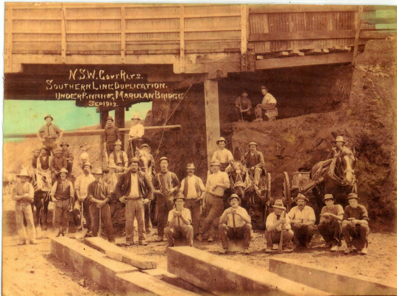
Expanding opening at overbridge carrying present day George St in preparation for track duplication. September 1913. (Berrima District Historical and Family History Society)
