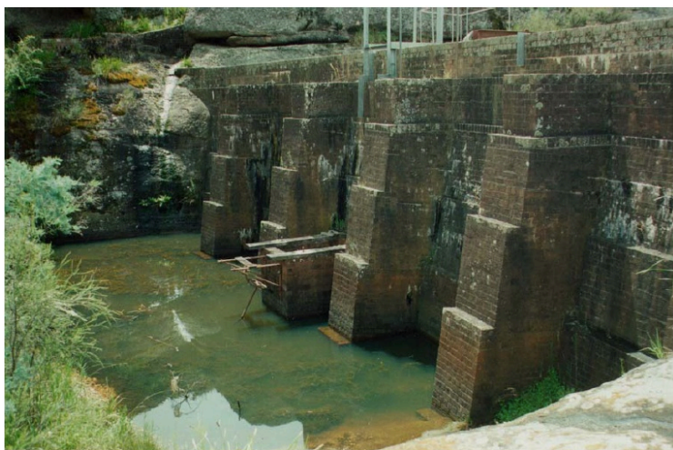
Part of downstream face of dam as it appeared in early 2010, showing evidence of remains of outlet works. (courtesy Rob Randazzo)
