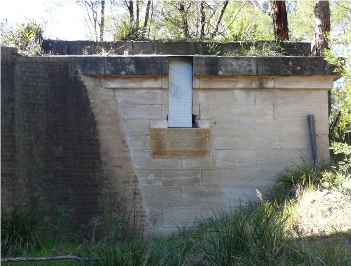
Eastern abutment of first railway bridge in July 2017 showing the slot and extra stonework for the central girder added in 1892.
