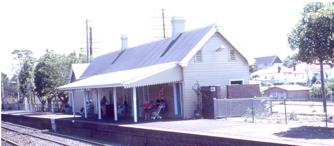
The timber building on the southbound platform on 26 th December 1977. The brick privacy screen protects the entry to the male toilet. The steel mesh fencing was typical of the 1960s and 1970s.
