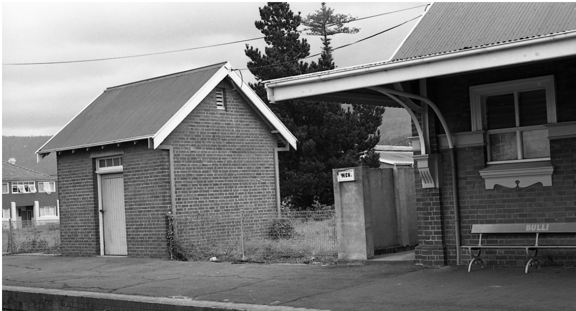
The rendered brick privacy screen in front of the entrance to the male toilet is unusual. Originally, a timber screen had been provided.
