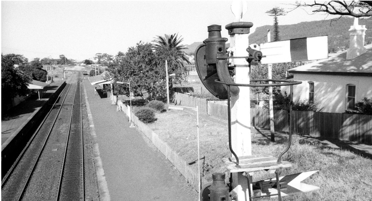
This photograph shows the Up Second Home signal for Bulli and the Up Inner Distant signal for Bulli Coal Siding . The 1885 approved residence for the Station Master is located to the right. It will be noted that the goods yard is much further to the south than it was in the single line days. Photograph No.466669 ARHS Collection, N. Munro, 24 th April 1984.
