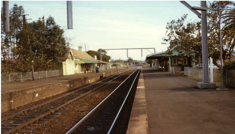
In this photograph, the overhead stanchions are in place, but the wires are not yet been hung. The vegetation on both sides of the rail corridor looks out of control. The platform surfaces appear in reasonable condition. Image No.026691c ARHS Collection, G. Dornan, 1 st October 1984.
