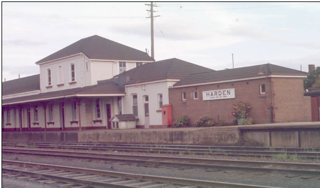
The unpainted structure dates from a time between 1946 and 1957 and possibly when the northbound platform was extended in 1954 at the southern end. The doghouse for two animals is located adjacent to the entrance to the then sitting room for refreshment room staff. Taken on 28 th May 1982.
