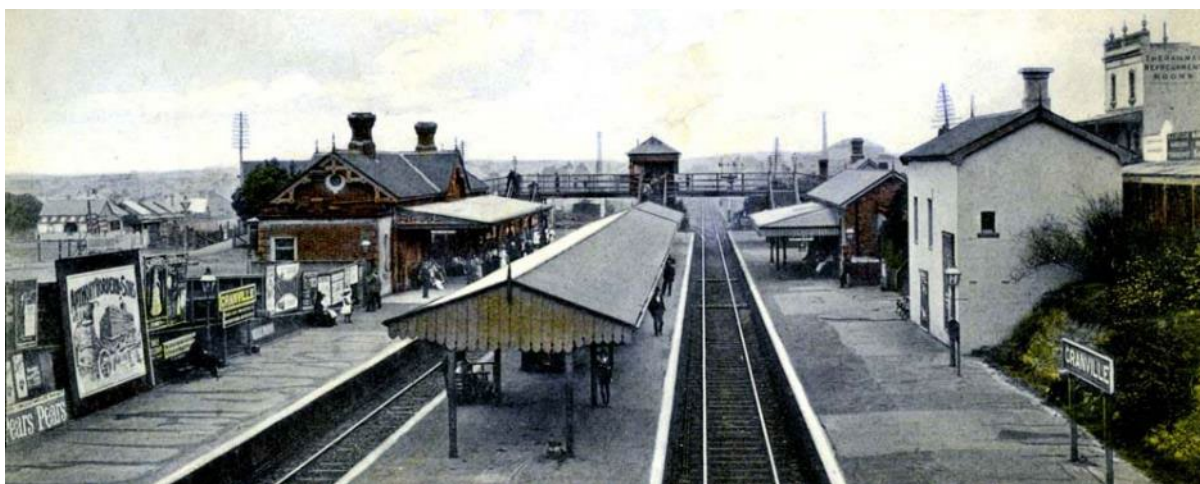
A colourised, printed postcard of Granville station. The similarity of the 1880 structure on the left to the Harden building is evident in the gabled roof, bulky chimneys, finials and transverse gables. SOURCE: Photograph No. 510137, ARHS Railway Archives.
