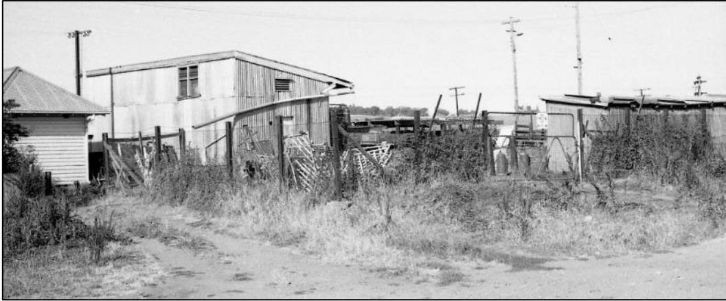
This photograph taken on 19 th January 1983 from Whitton Lane East shows the level of amenities that per way and signalling staff used prior to their relocation into the vacant space of the former refreshment room in the 1970s and 1980s.
