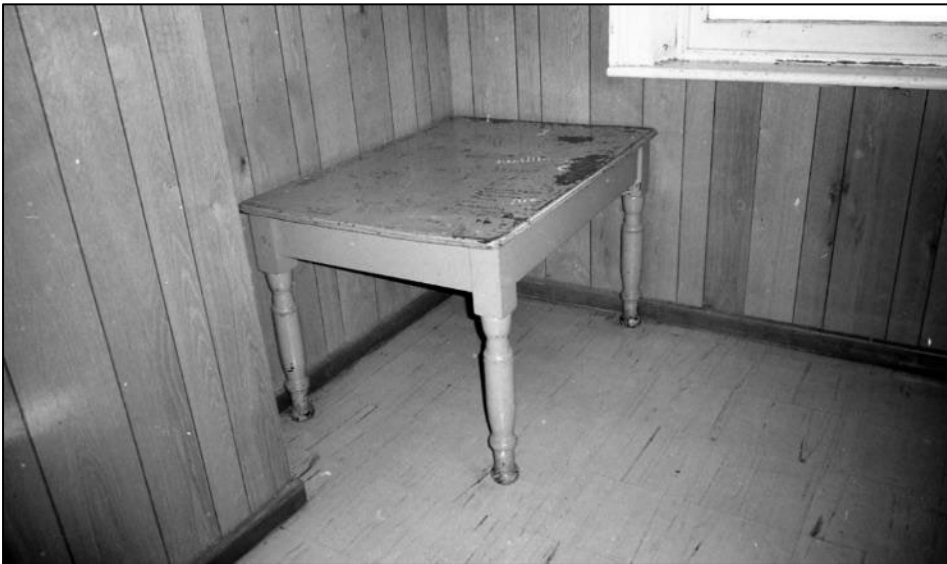
Besides the timber bench, the only other piece of furniture in the ladies' waiting room was a table. The fake timber wall panelling has been used to cover the former fireplace. Taken on 23 rd August 2000.
