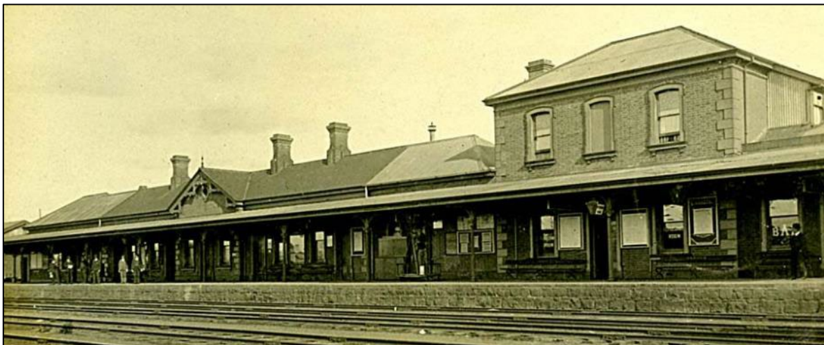
This photograph shows the building on 14 th May 1909. The transverse gable in the middle of the roof identifies the entrance to the platform from the general waiting room and station forecourt. SOURCE: Photograph No. 510544 ARHS Railway Archives
