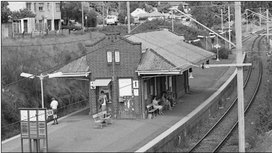
The above photograph shows the city bound side of the station looking towards Kingsgrove. The original corrugated asbestos cement roof sheeting is in place. The lady sitting on the seat closest to the camera marked the position of the approved but not built open-sided general waiting room. Above the lady's head is the original ticket window. The photograph was taken on 3 rd March 1984.
