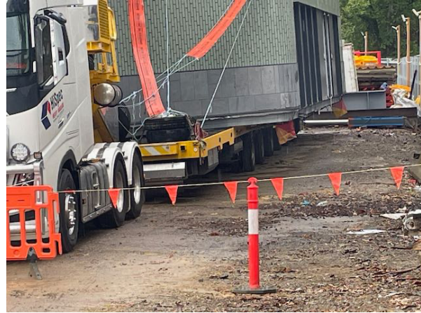
Prefab building on low loader in Surrey Park.
