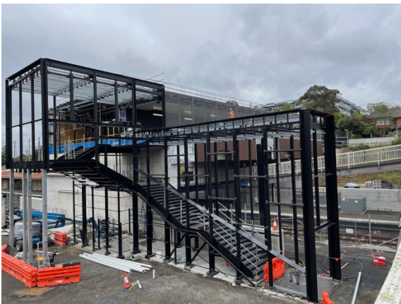
Greensborough Station from Footbridge looking across to Shops South Direction 2022|122 GWa
