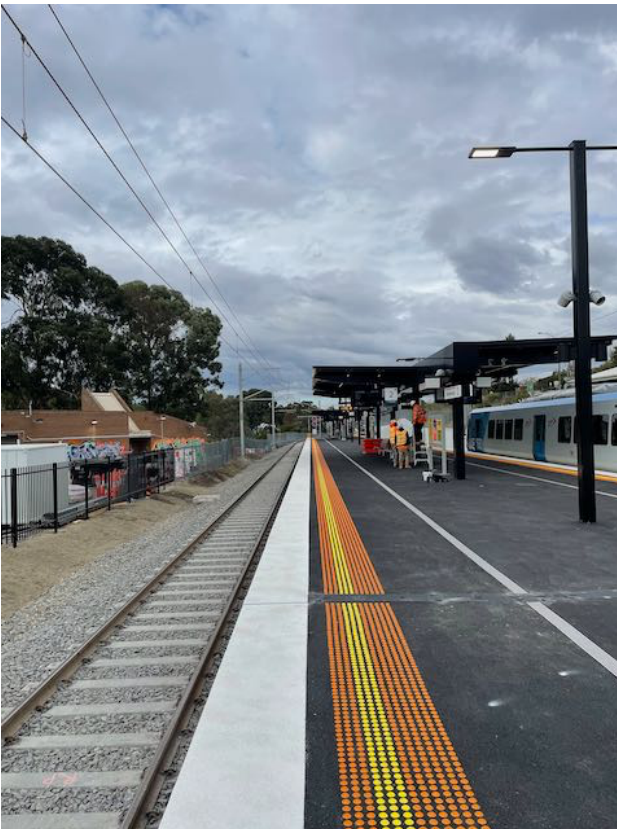
Greensborough Down Platform in Down Direction showing workers on 2 nd Day of Opening.
