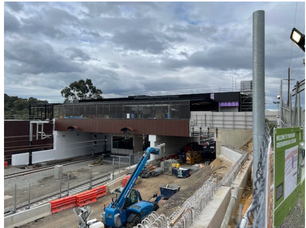
Greensborough Station looking in Down Direction at new Concourse from Footpath.
