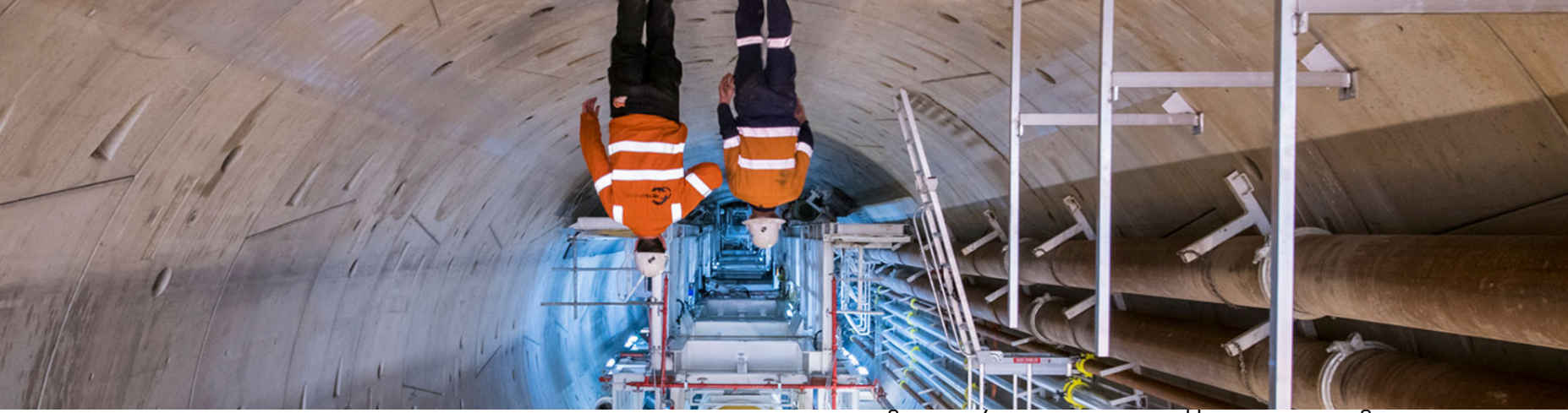
Arden Station showing framework to support the arches as they are being installed.
