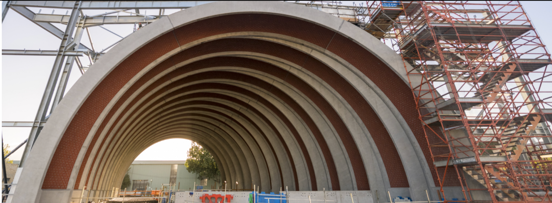
Arden St Station Entrance arches completed. Photo by GWa
