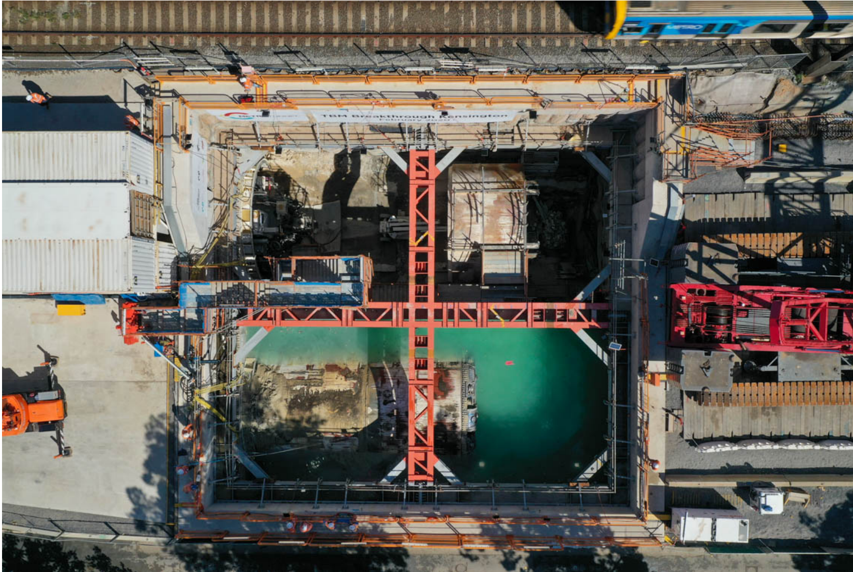
Western Portal overhead view showing Cutting Heads about to be retrieved & taken back to Arden Station site by truck for reuse on next tunnel to be bored.
