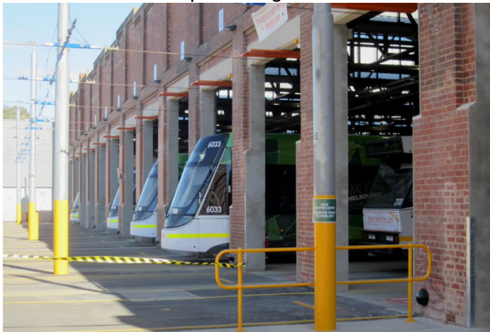
The new Improved Preston Depot showing E Class Tram Noses peeking out.
