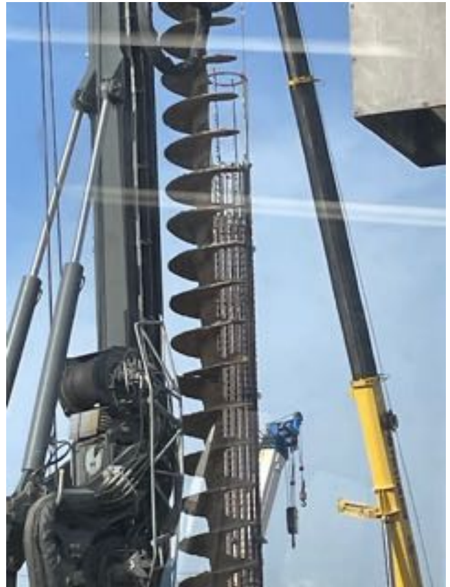
Drilling Rig on Glenhuntly Road 20230522 GWA Photo
