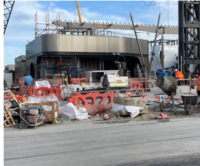
Glen Huntly Station Buildings looking in Down Direction 20230713 GWA Photo
