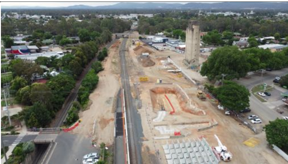
The new seal on the platform shows where the now filled in underpass was located, looking in Down direction towards Benalla. AB Photo
