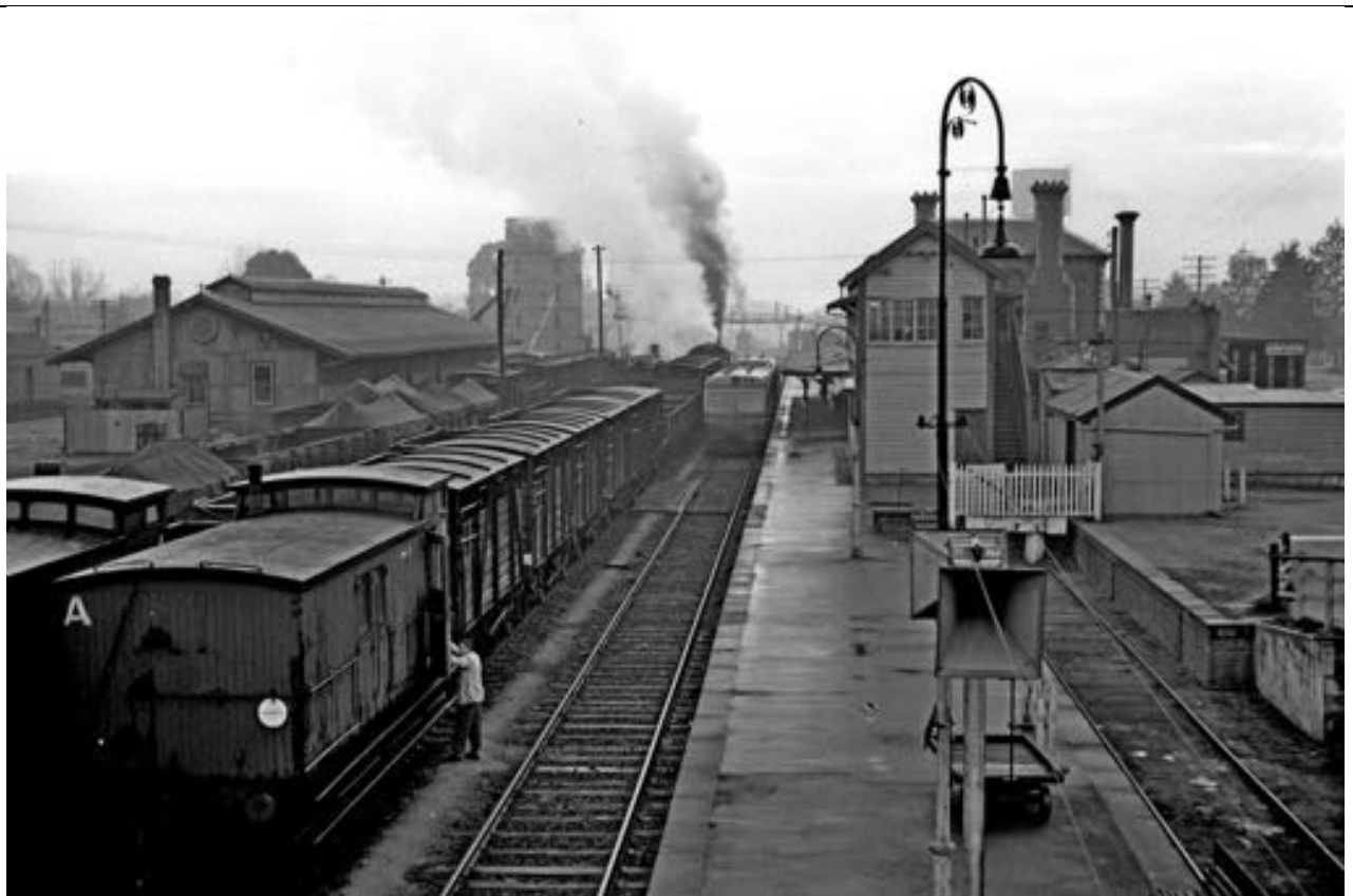
This 1956 photo is displayed in the Wangaratta Waiting Room. It shows the 7.35 am 280 HP railcar, an R class hauled good in No. 2 road, the Peechelba goods in 3 road and a shunting loco (possibly a D3 at the far end of the yard. The new but now installed, but covered in, pedestrian subway is close to the location of the old fashioned loud speaker. AB Photo
