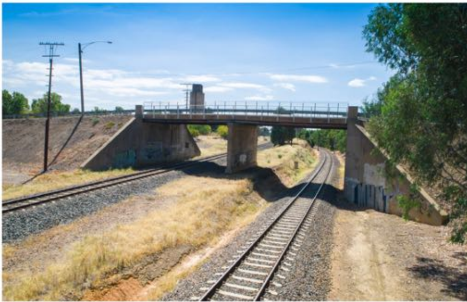
Existing Green Street bridge.
