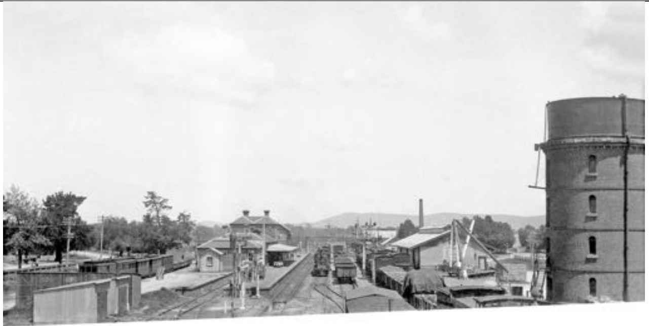
This shows the narrow gauge carriages on the head shunt and a man on the carriage roof, presumably filling the small water tank located in the top of the carriage. It also shows the pair of water cranes for watering double headed locos. Unfortunately the photo does not show the twin ash pits, that other photos I have, do show. This photo as far as I know has never been published. Supplied by AB.
