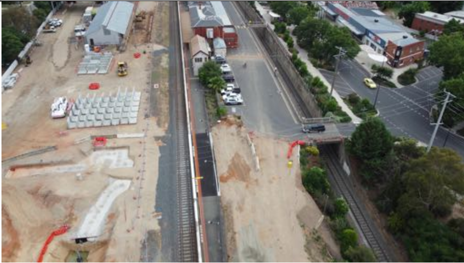
The new seal on the platform shows where the now filled in underpass was located, looking in Up direction towards Wodonga. AB Photo
