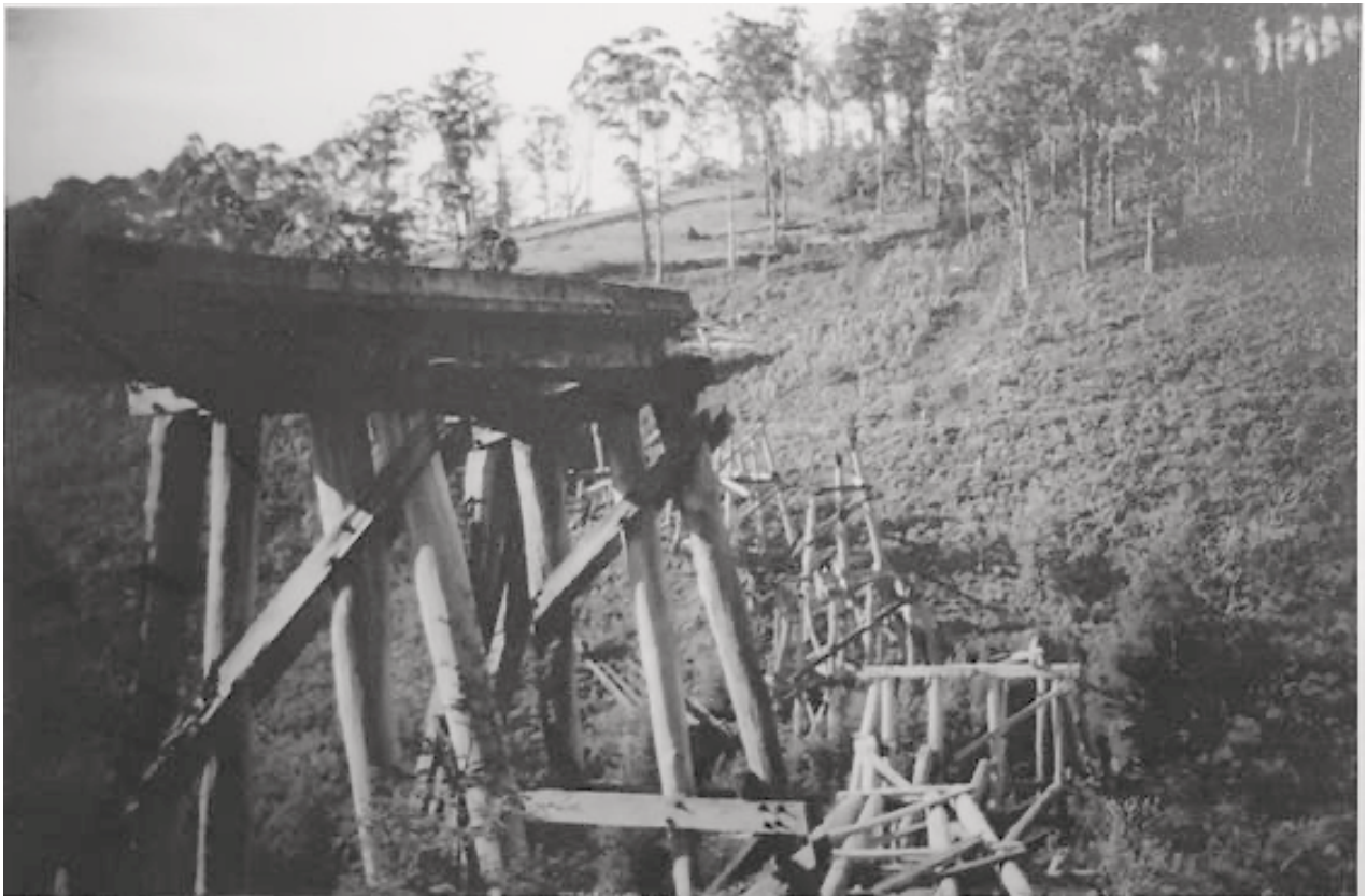
Noojee railway line closed 1954, 1962 photo of burnt trestle bridge Noojee
