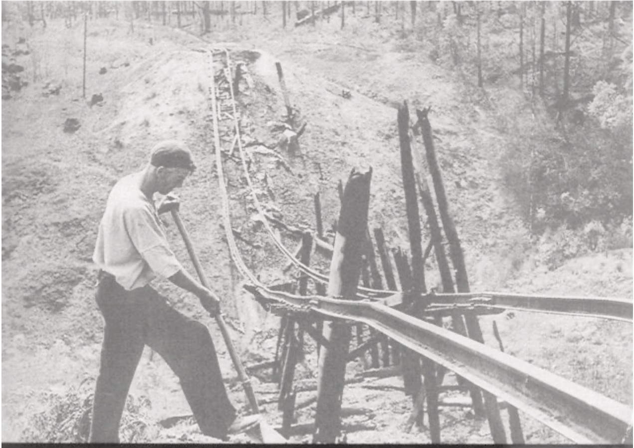
Noojee Line destroyed Trestle Bridge 1939 01 13
