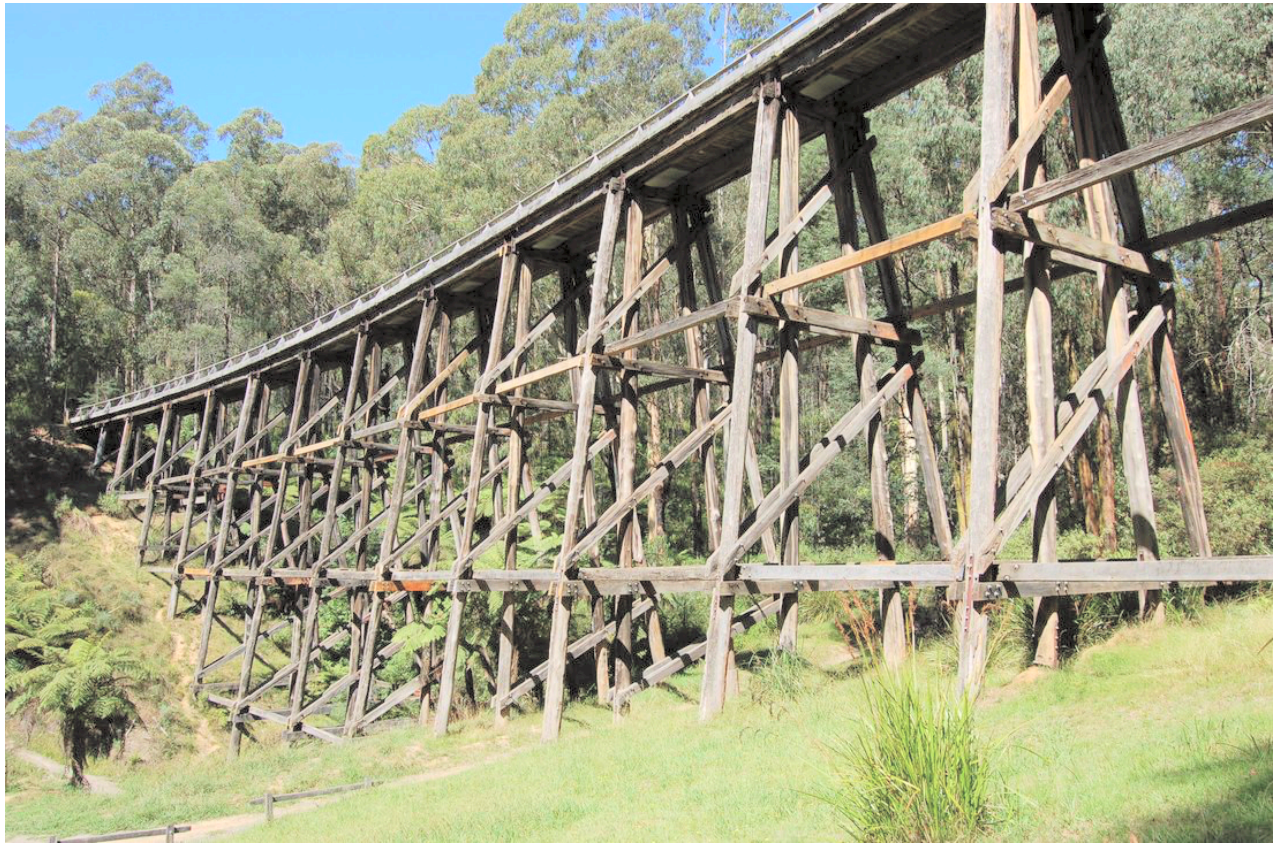
Noojee Trestle Bridge Rail Trail_001 VicScreen
