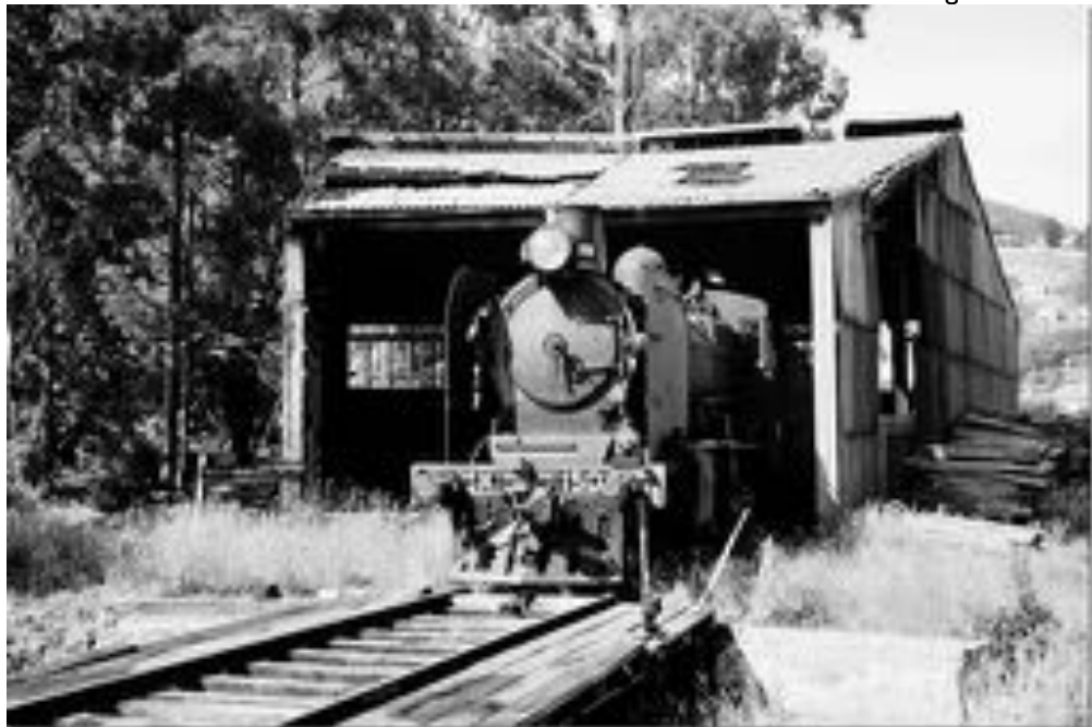
K150 just about inside a very dilapidated Engine Shed, note shed on LHS, one road & Chimneys missing shown on next image 19621216 Bob Wilson Image
