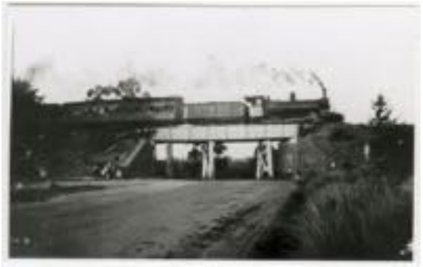
Photograph of new steel railway bridge on Maroondah Highway, Lilydale with steam engine and carriages crossing for initial testing. Unknown Image.
