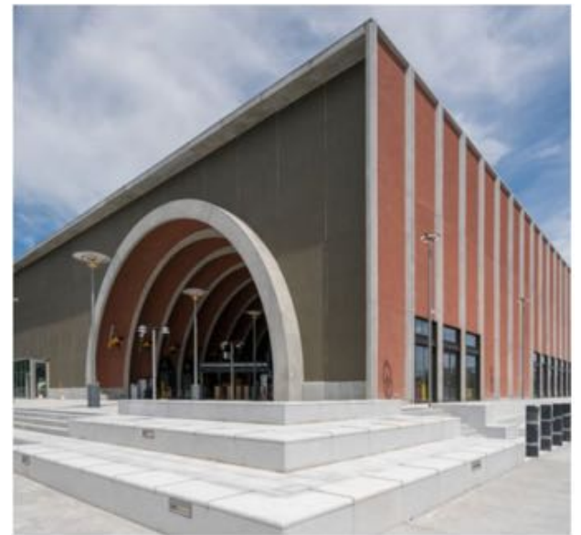
Arden Station from Arden St. Image from <bigbuild.vic.gov.au>
