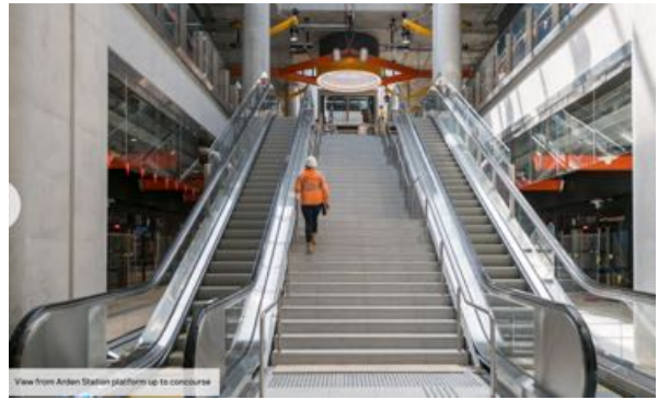
Arden Station Platform looking up to Concourse. Image from <bigbuild.vic.gov.au>
