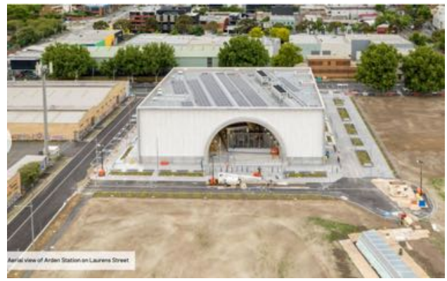
Aerial view of Arden Station on Laurens St. Image from <bigbuild.vic.gov.au>
