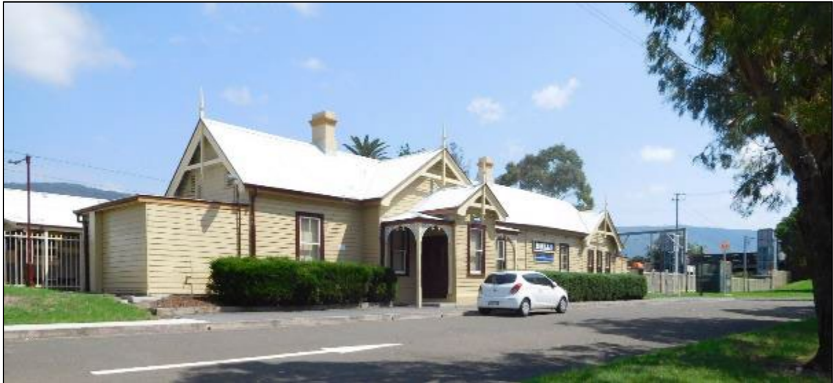
This photograph shows the rear of the building at Bulli on 29 th January 2000.
