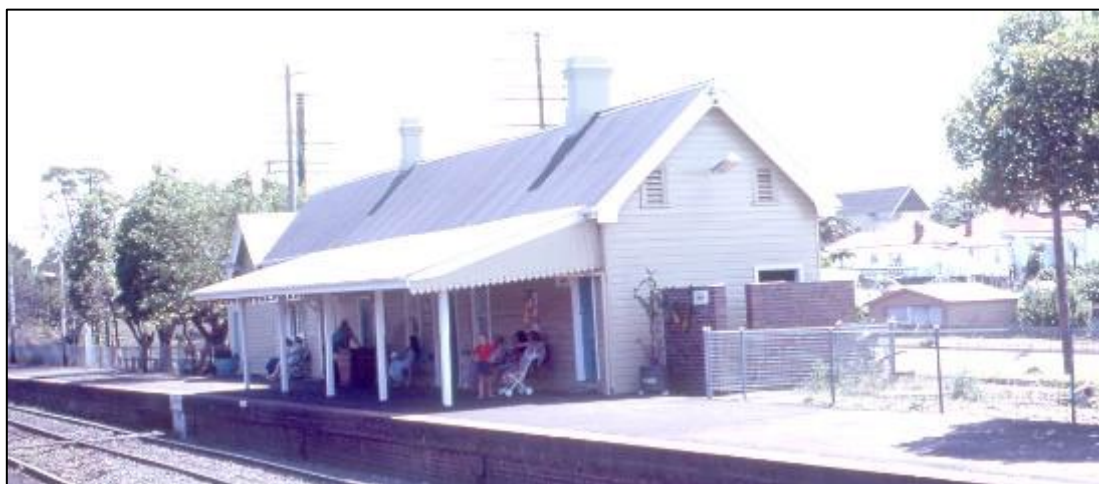
The timber building on the southbound platform at Bulli on 26 th December 1977. The brick privacy screen protects the entry to the male toilet. Previously, toilets were located in a separate pavilion. The steel mesh fencing was typical of the 1960s and 1970s.
