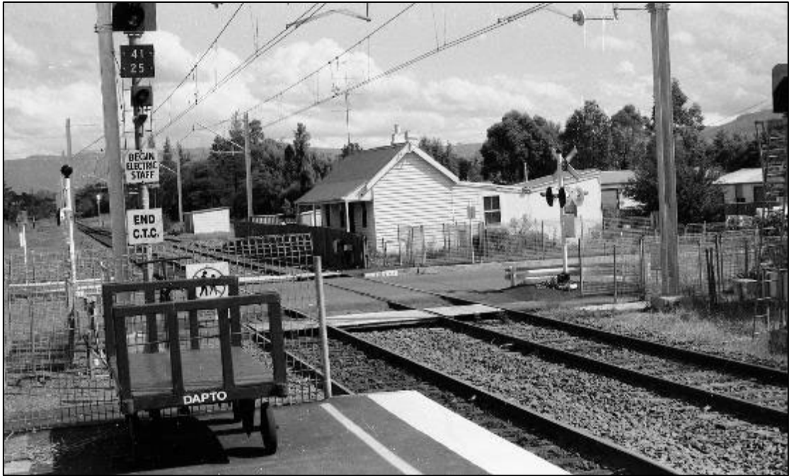
The above photograph, taken on 26 th December 1977, shows the timber gatehouse at the southern end of the platform
