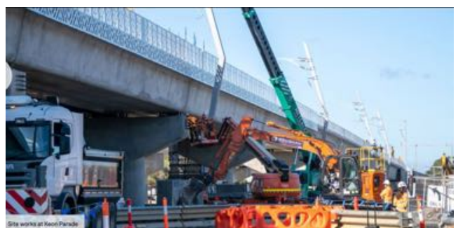
Site works at Keon Parade. Victoria's Big Build.
