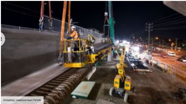
Installing L Beams at Keon Parade. Victoria's Big Build.
