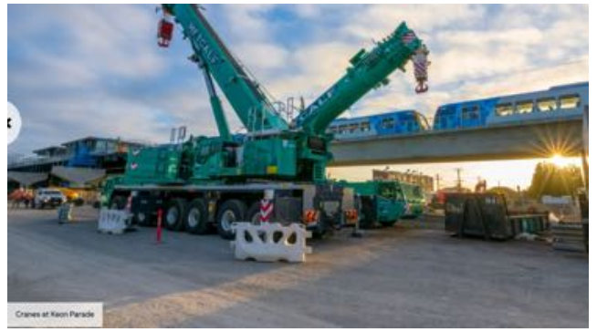
Cranes at Keon Parade. Victoria's Big Build.
