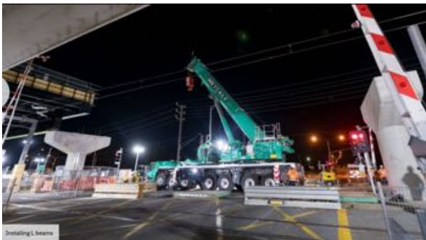
Installing L Beams. Victoria's Big Build.
