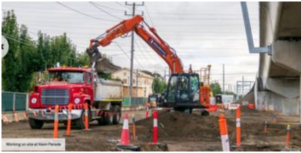
Working on site at Keon Parade. Victoria's Big Build.
