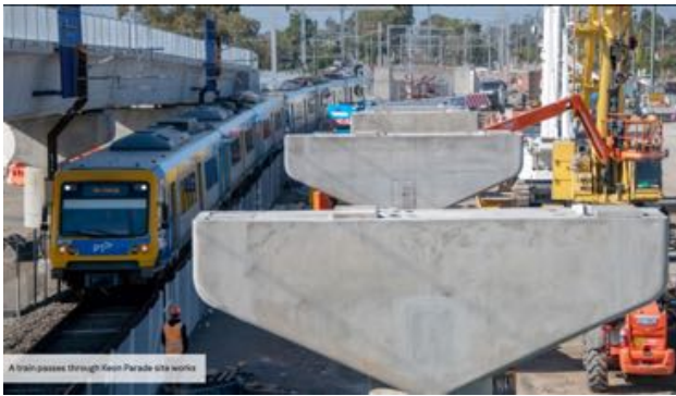
A Train passes through Keon parade Site works. Victoria's Big Build.
