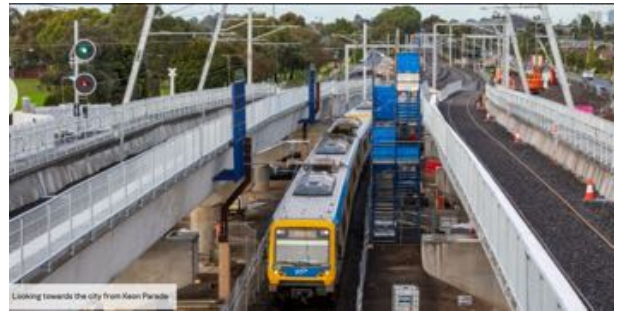
Looking towards the City from Keon Parade. Victoria's Big Build.
