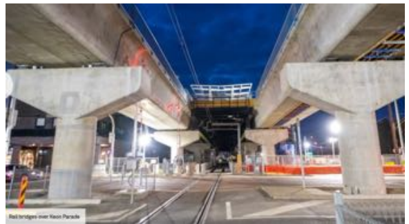
Rail Bridges over Keon Parade. Victoria's Big Build.
