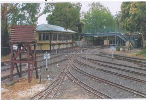
Diamond Valley Railway B signal box, main station and tracks coming from the sheds and the main line. 5.12.2015 (Peter Charrett)
