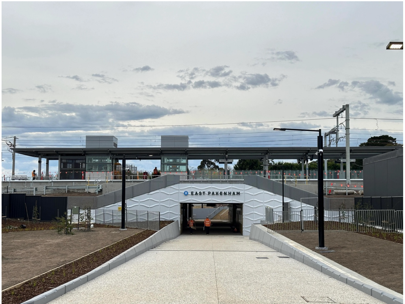
East Pakenham Station day before Opening 2 nd June 2024. By East Pakenham oh yeah, it's finally here - https://www.flickr.com/photos/200812091@N04/53765874060/ , Public Domain, https://commons.wikimedia.org/w/index.php?curid=149018474
