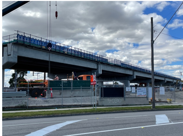
Elevated Rail viewed from Main Road Pakenham 20230316 GWa
