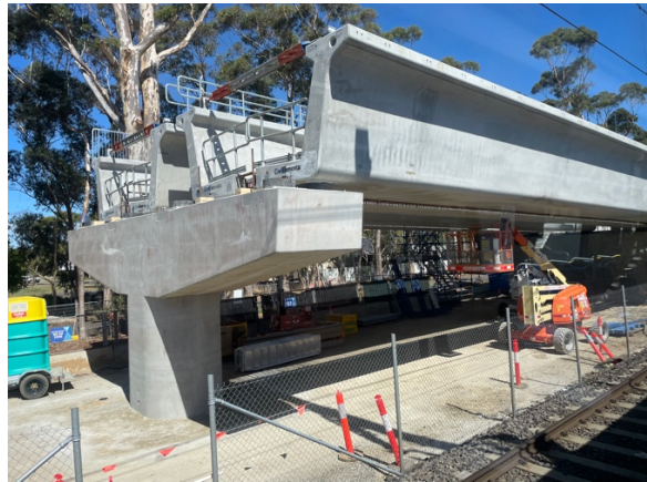
Crosshead & L Beams 20230316 GWa
