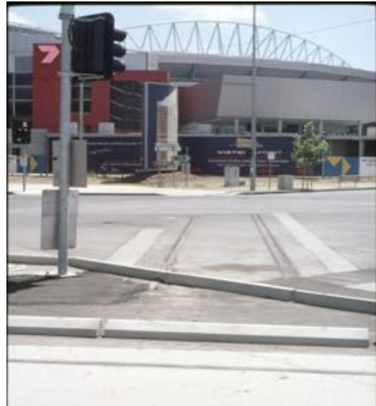
Where track crossed Harbour Esplanade 20021226 WL
