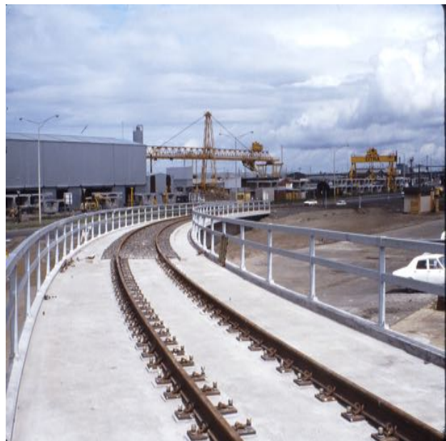
Webb Dock Rail Link Yarra River Bridge south end now used for Pedestrians & Cyclists 19850918 WL
