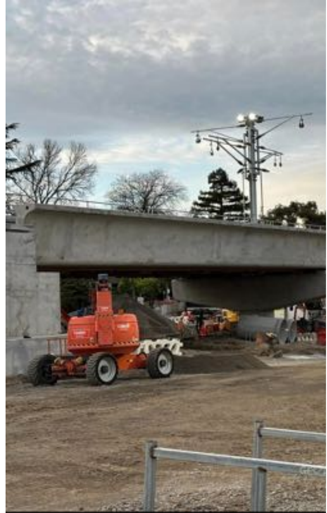
Croydon no overhead 20260627 Facebook Croydon & Ringwood Level Crossing Removal Updates Group
