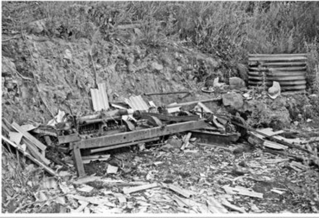
1944 - remains of the car engine and pulleys (John Thompson)
