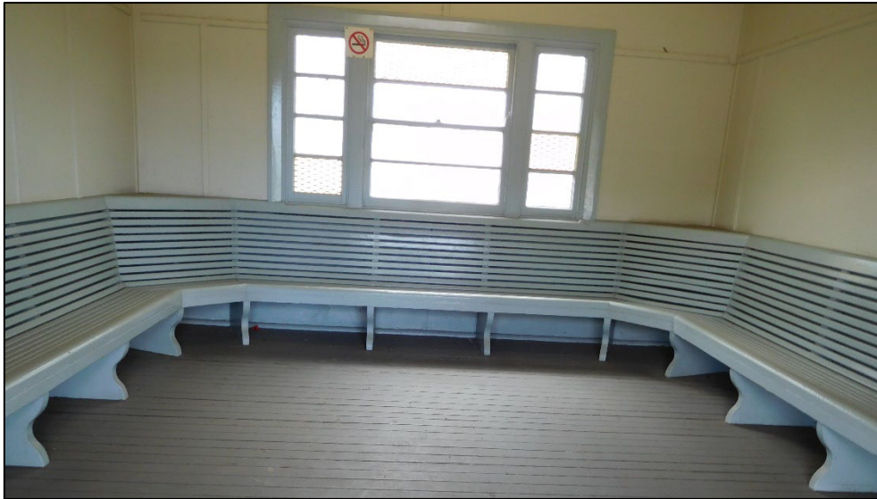
One of the hallmark aspects of the station is its original seating in both general waiting rooms. This image shows the widest room in the building on the northbound platform with the multi-slat, timber seats, which were typical of the 1930s. The image was taken on 3 rd March 2021.
