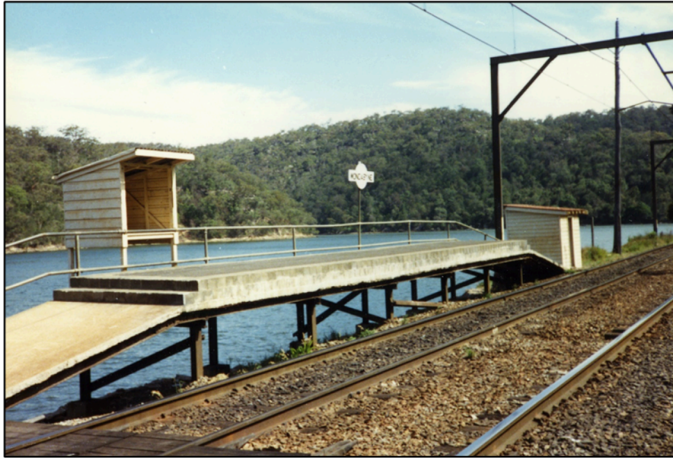
This 1985 photograph shows the 1943 waiting shed off the end of the southbound platform and the parcels box dating from the 1960s. The Department of Railways issued a standard plan in 1963 for a parcels box and 20 examples are known to have existed in parts of the rail network in rural and regional areas. SOURCE: Photograph No. 002796E, ARHS Railway Archives.
