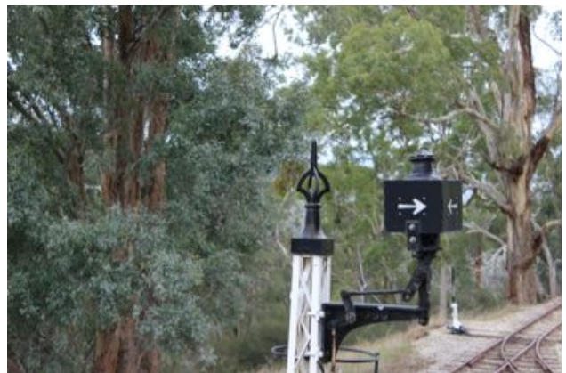
Out on the track on the way to the Summit showing Point Indicator at KMR. GWa pic 20140419
