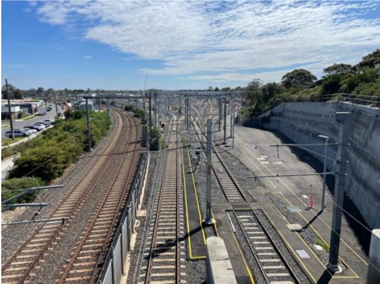
From the Road Bridge on the Up side of Kananook Station 20241016 GW image.
