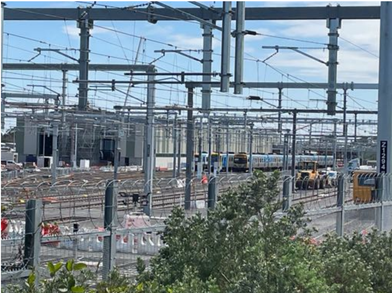
From Wells Road looking across the Stabling Yards to the 2 Road Maintenance Shed. 20241016 GW image.
