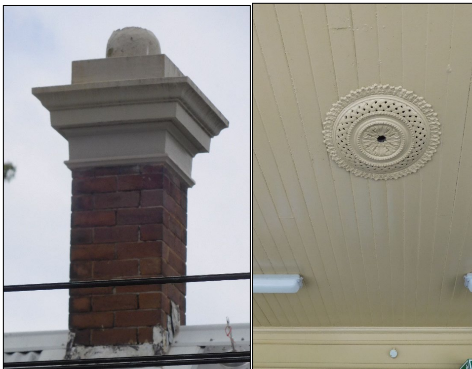
These two images show decorative elements. On the left is the chimney with corbelling (i.e. different levels of moulding) and a remnant of the terracotta pot. On the right is the ceiling rose on the overhead booking/parcels office. Its role was to evacuate fumes from kerosene or gas lamps. Similar roses were used in the ceilings of the 1909 platform building.
