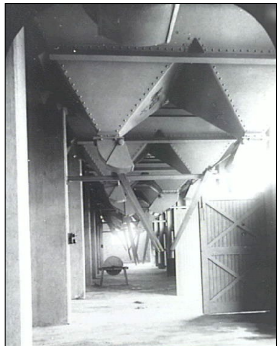
This photograph shows the bins underneath the two tracks. The long handles open and close the outlets. The gravel discharged into road vehicles beneath the bins. SOURCE: Photograph No. 1810 Ku-ring-gai Library Local History Collection.
