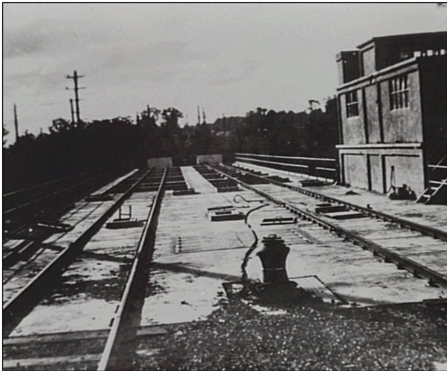
The photograph on the left, taken about 1928, shows the two sidings with the bins at the far ends of the tracks. The capstan to move the rollingstock is in the foreground. SOURCE: Photograph No. 1995 Ku-ring-gai Library Local History Collection.
