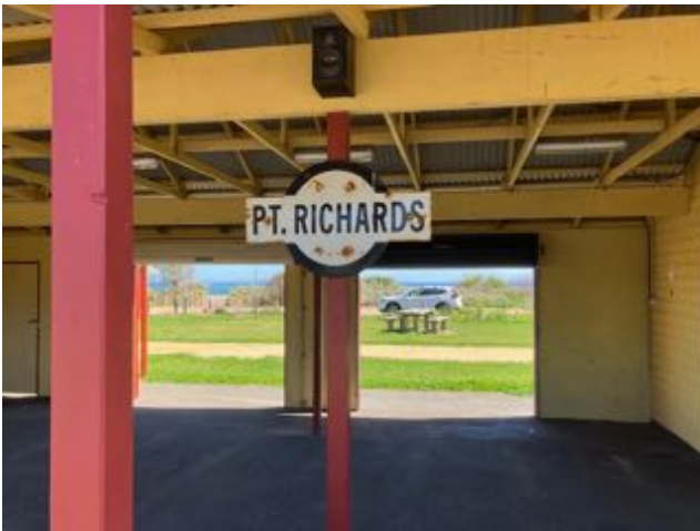
Point Richards Station Sign JR 20241009
