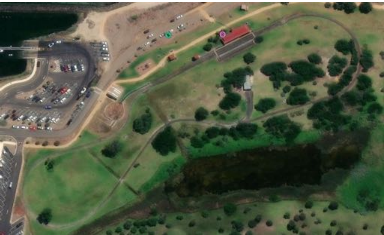
Aerial View of PMR showing Station & Loco Prep Area & Turntable Apple Maps 2024-12-24
