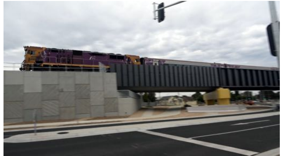
STH GEELONG - up pass on bridge over Fyans St 202411
