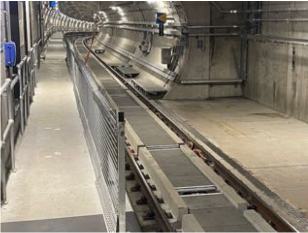
Arden Station Open Day showing tracks and anti-derail Concrete blocks between tracks 20250830 GWa Pic
