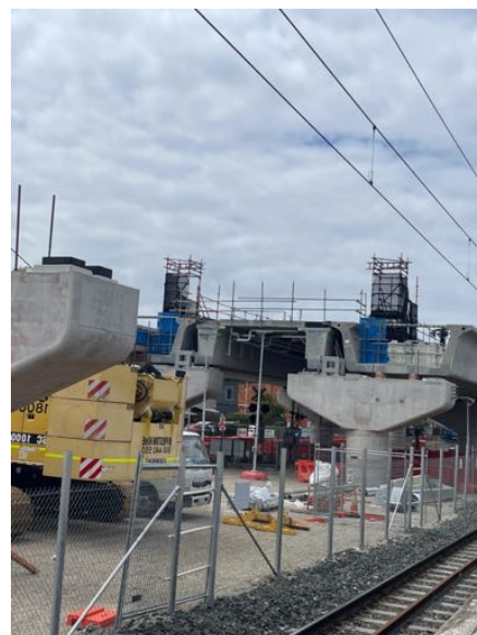
Platform construction between two elevated tracks looking in Down Direction 20260104 GWa
