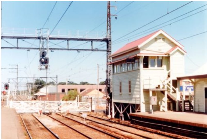
Signal box & gates at Bear St level crossing soon to be replaced with booms & color light signals 17-03-1986 JS Image
