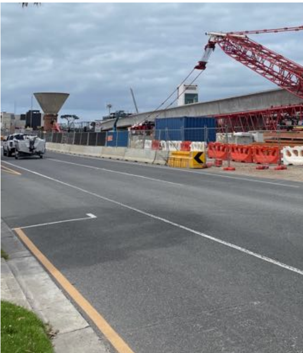
Steam Era Water Tower showing how close to new elevated tracks 20260104 GWa
