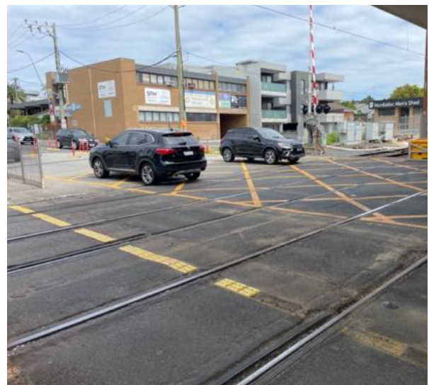
McDonald Street LX at Up End of Mordialloc Station, showing 3 old tracks, only track closest to black cars in use now, looking NW 20260104 GWs Pic
