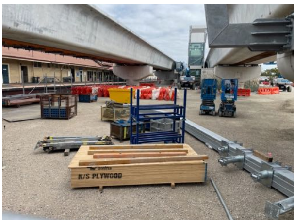
Looking between new elevated tracks to lift shaft and original Platform 1 on LHS of pic 20260104 GWs Pic
