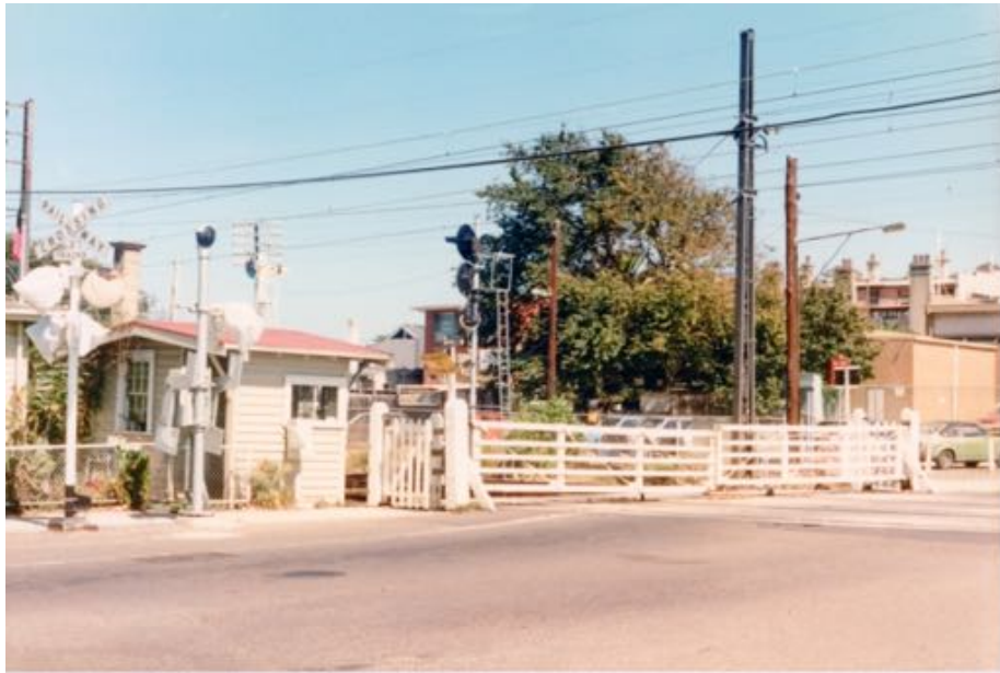
Gate house & hand operated gates at McDonald Rd level crossing soon to be replaced with booms & color light signals 17-03-1986 JS Image
